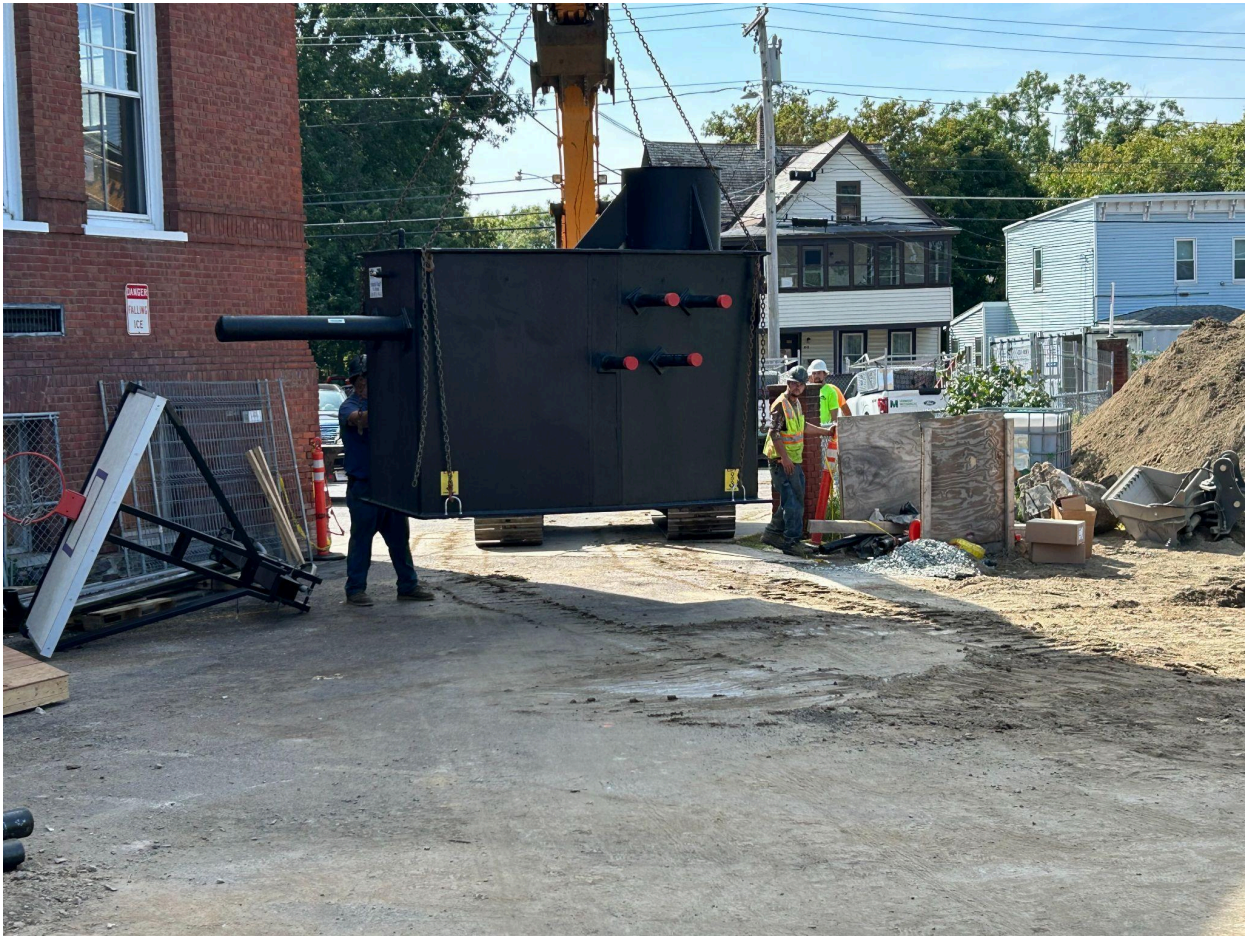
A picture showing the new geothermal vault being moved from the delivery trailer into the site.
