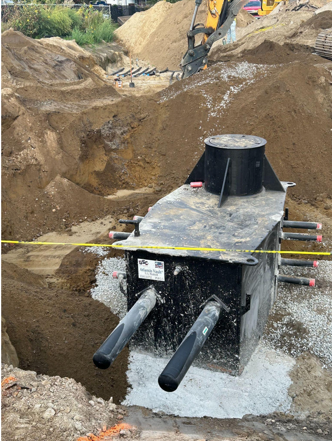
A picture showing the final resting place for the geothermal vault. In the foreground, you can see the geothermal piping heading in the direction of the vault. Manosh is in the process of extending and attaching the piping to the new vault.
