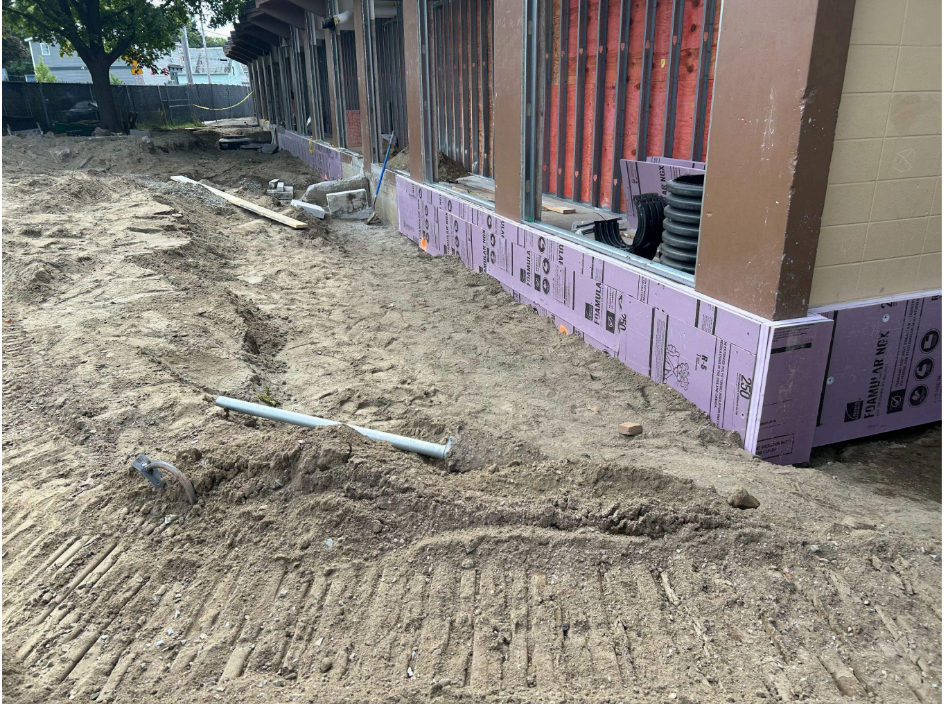
This picture is showing the installation of insulation on the Walnut Street side of the building against the foundation.
