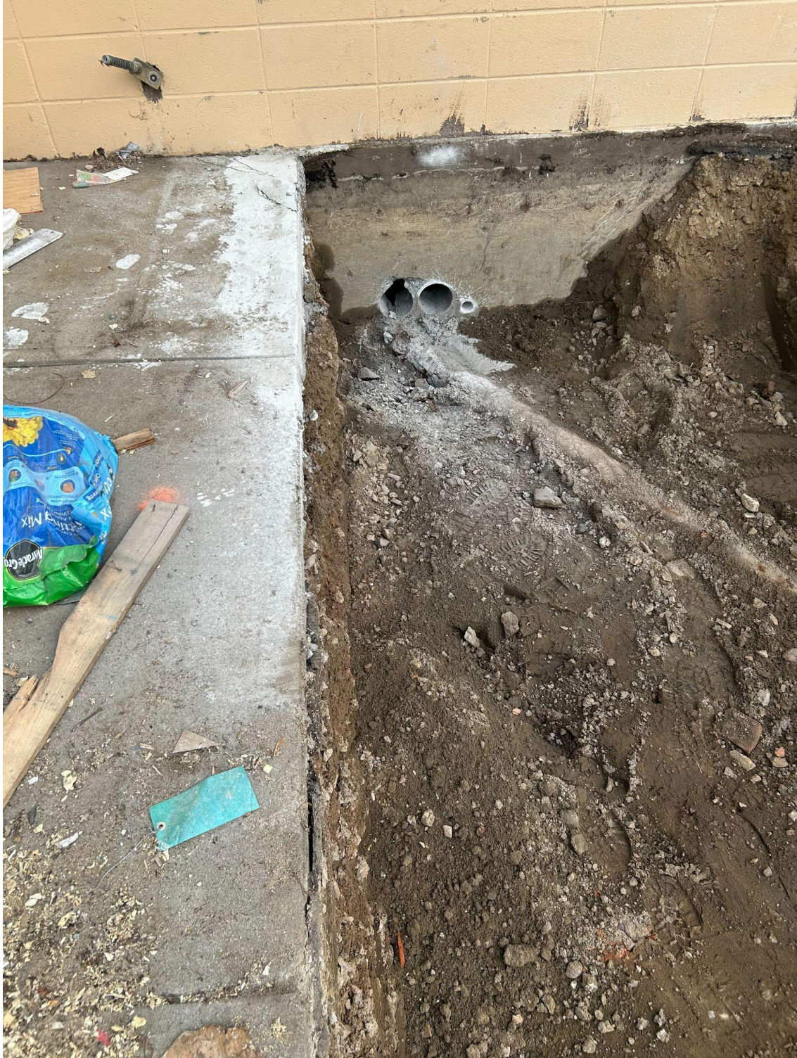
Picture showing the existing concrete foundation wall being cut, so that new electrical conduits can be installed from the new transformer into the building and to the existing Electrical Room in the 1965 wing of the building.
