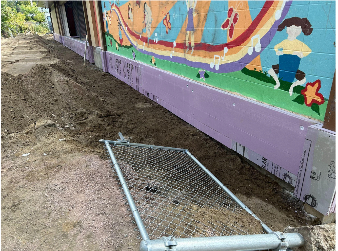
This picture shows the installation of insulation on the back side of the building against the foundation.
