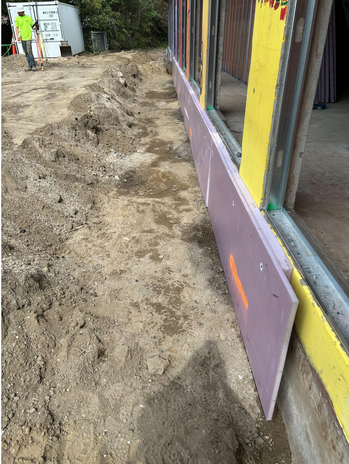
This picture shows the installation of insulation on the Manhattan Street side of the building against the foundation.
