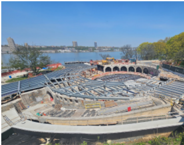
New steel structure
