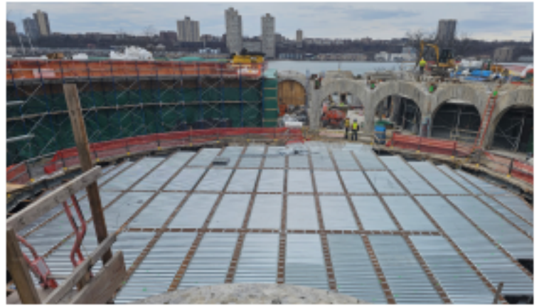
Formwork for center fountain on plaza level
