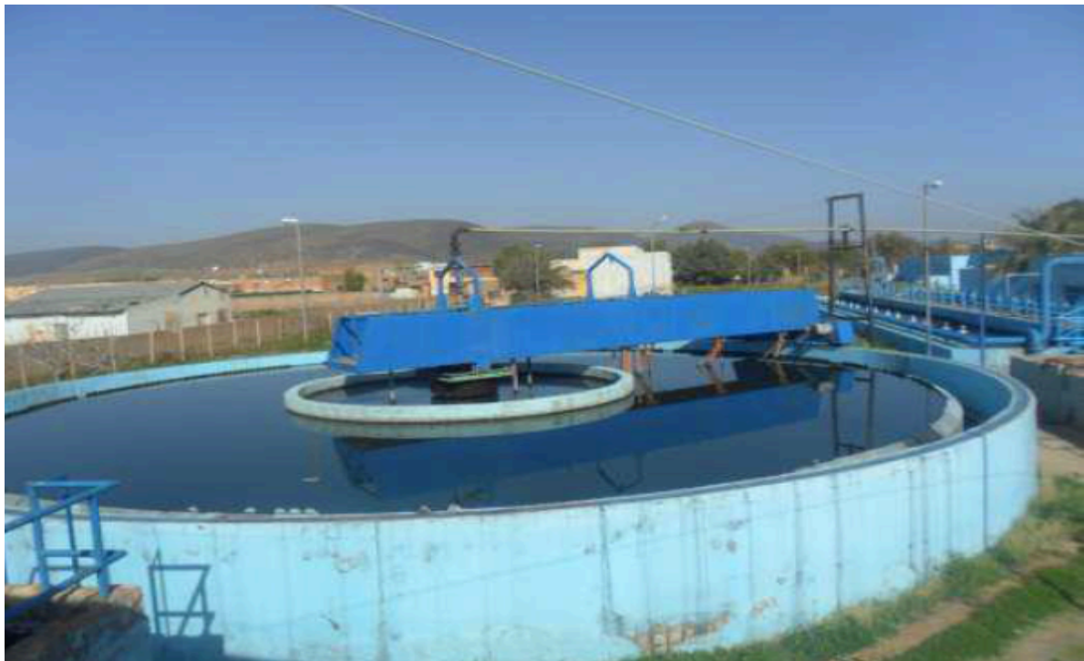
Figure 4. Clarifying flocculator.
