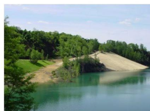
View of the erosion control matting installed on a 2:1 slope after cutting and regrading.
