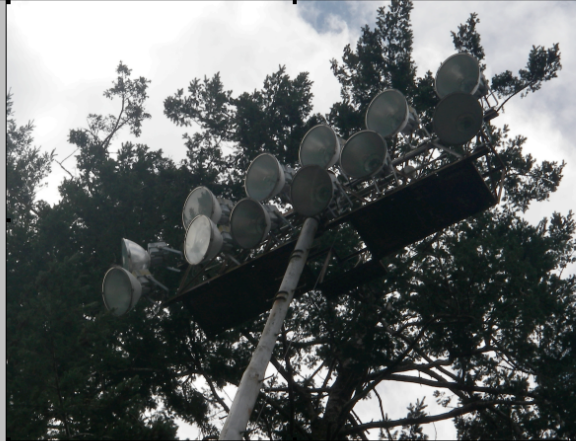
Fig 2: Arcata Sports Complex. Note fixture/reflector configuration. Vendor: Musco Lighting
