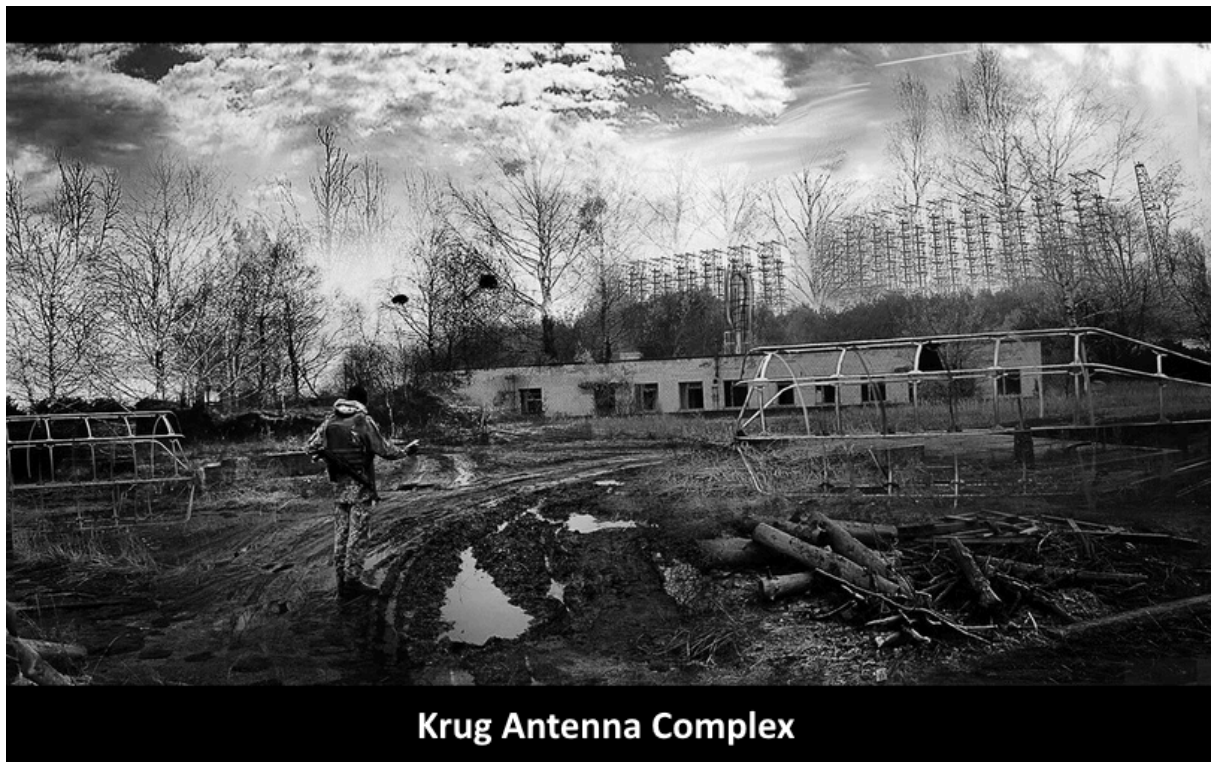
Krug Antenna Complex with fallen antennas
