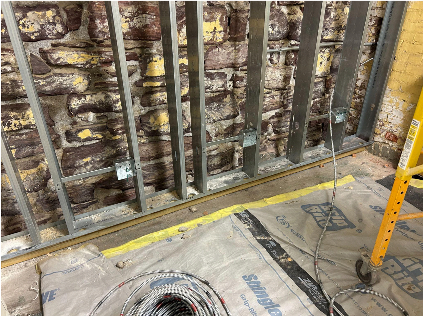
The electrical contractor is roughing in for the electrical outlets and data outlets in the B09 classroom in the 1904 wing of the building.
