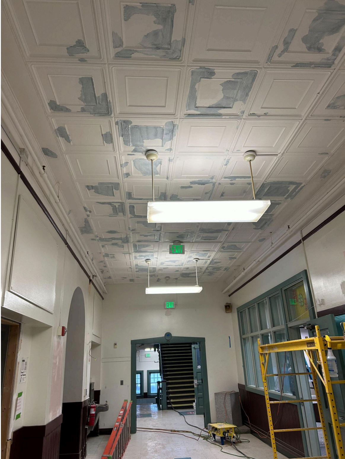
The ceiling of the First Floor in the 1904 wing of the building, where the painting contractor has removed the old paint and has applied a primer for now.
