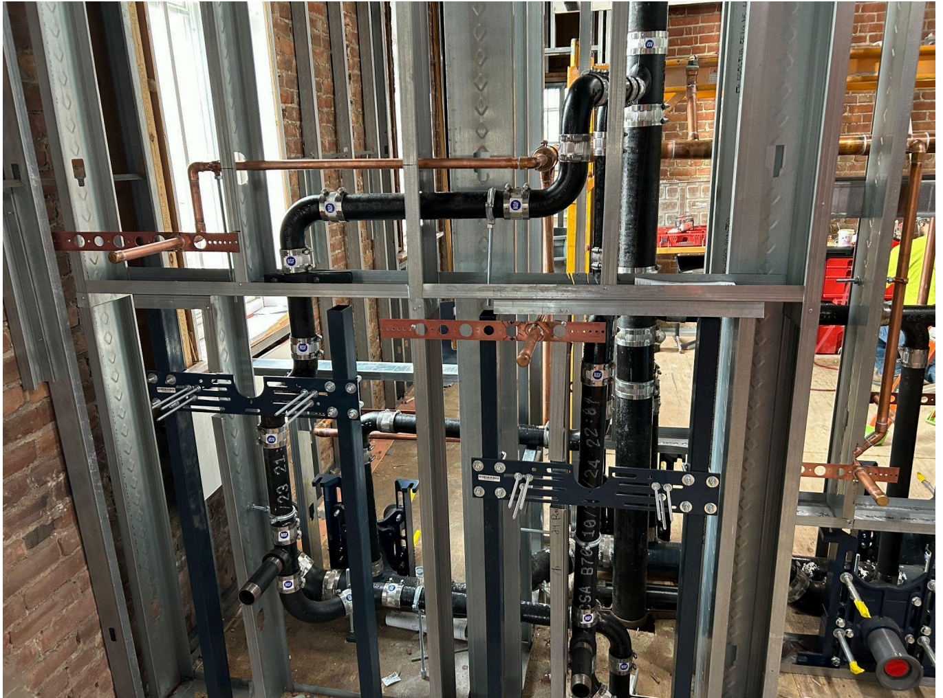
A different picture of the domestic water being installed for the gang bathroom in the 1904 wing of the building.
