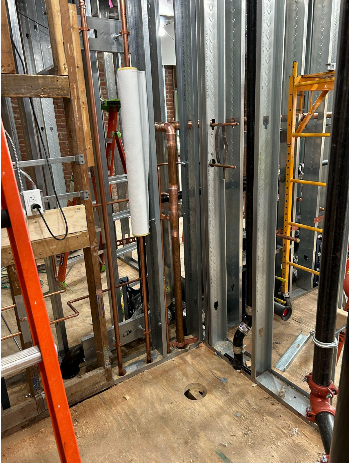
The new domestic water piping is being installed this week for the renovation of the gang bathroom on the second floor of the 1904 wing of the building.
