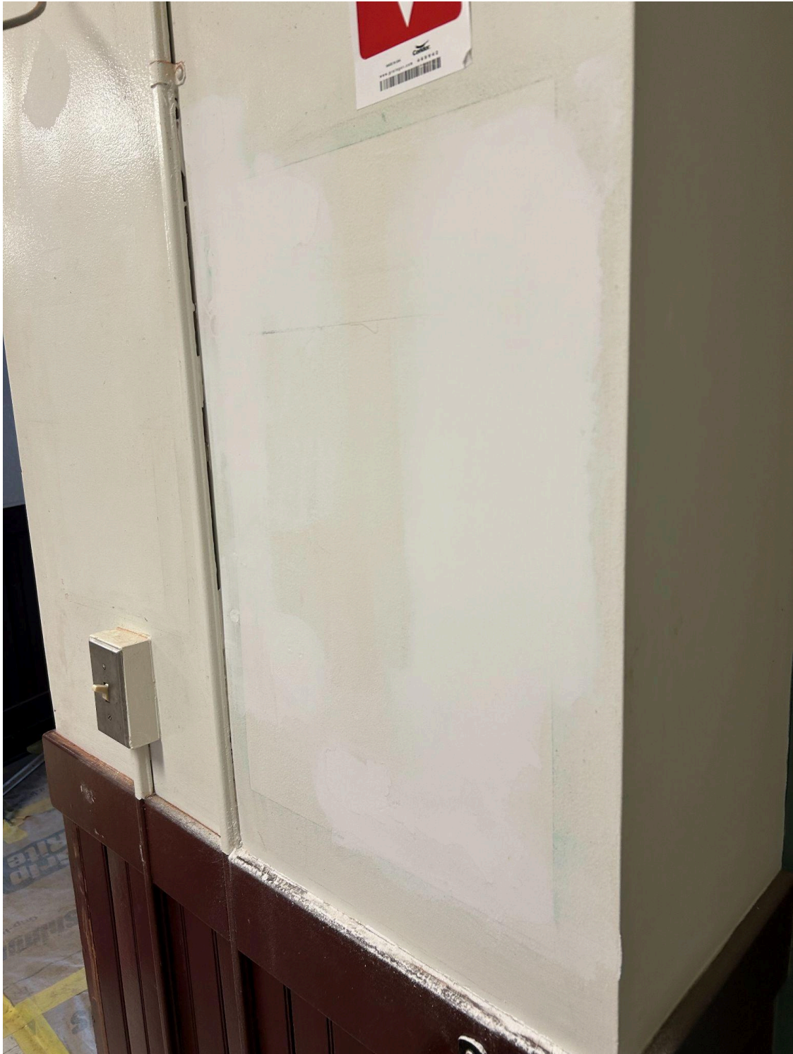
Another picture showing that the painting contractor is prepping the wall to be smooth, so that it looks like no holes have been there.
