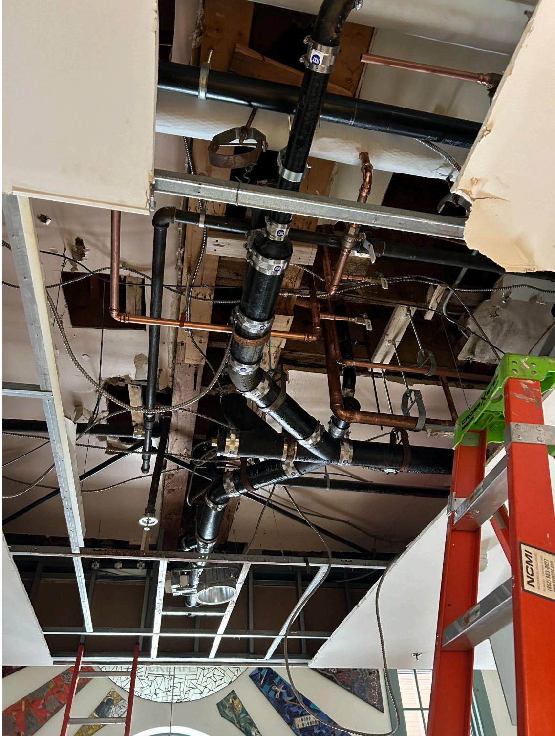
A picture showing the installation of new sanitary sewer piping for the gang bathrooms on the second floor in the 1904 wing of the building.
