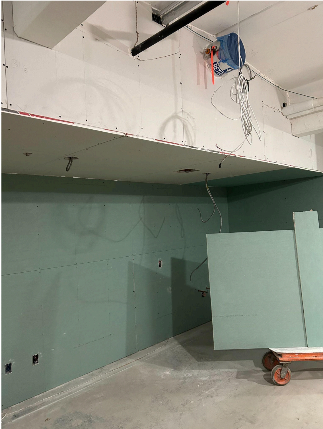
Sheetrock being installed on the walls and soffits in the classrooms of the 1965 wing of the building.
