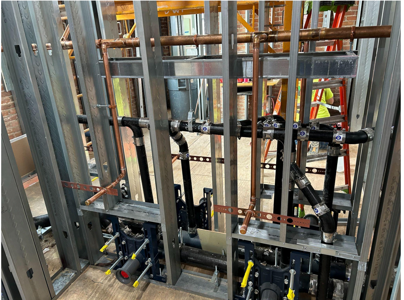
Another picture of the domestic water piping being installed for the gang bathroom in the 1904 wing of the building.
