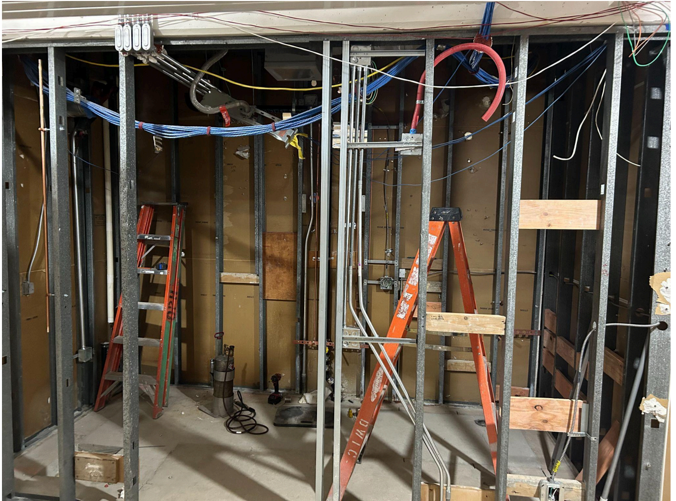
The Laundry room in the 1965 wing of the building is getting roughed in for the plumbing and electrical for the renovation of this room.
