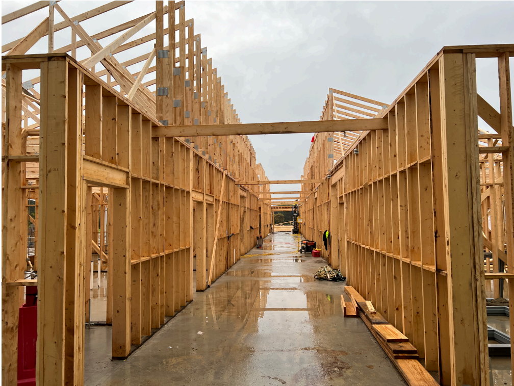
Upper Elementary Hallway
