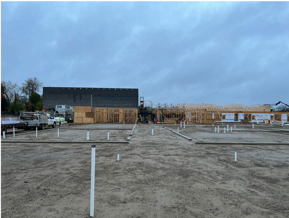
Main Corridor from Lower Elementary Wing to Upper Elementary Wing
