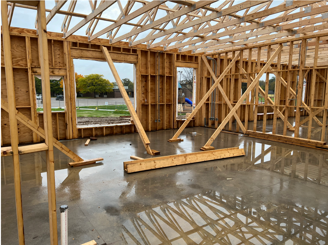
3rd Grade Classroom (Internal View)
