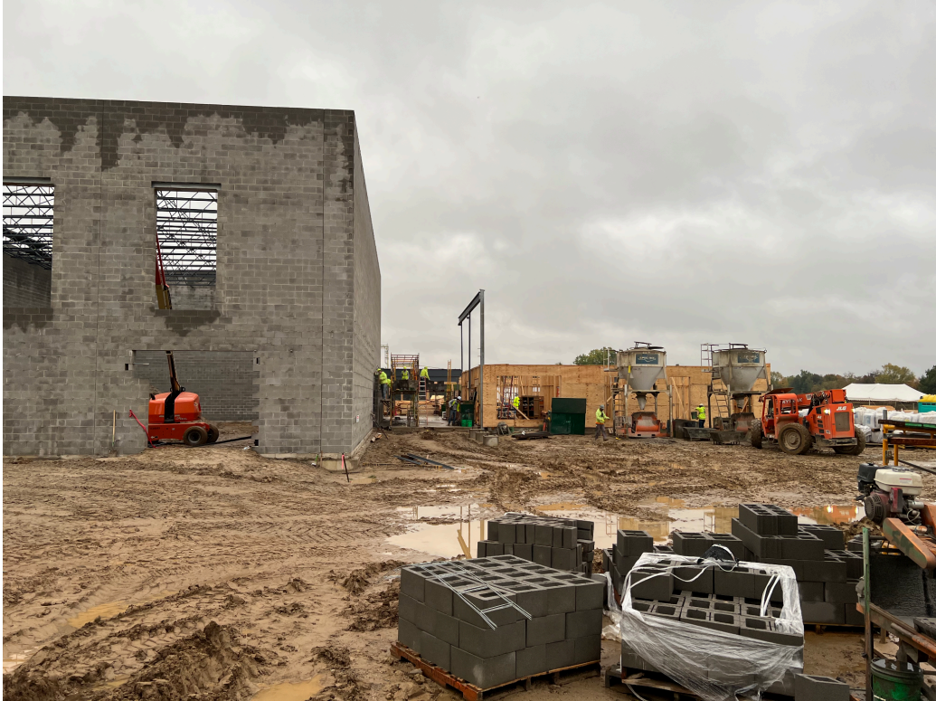
Main Entrance (Outside Looking In)
