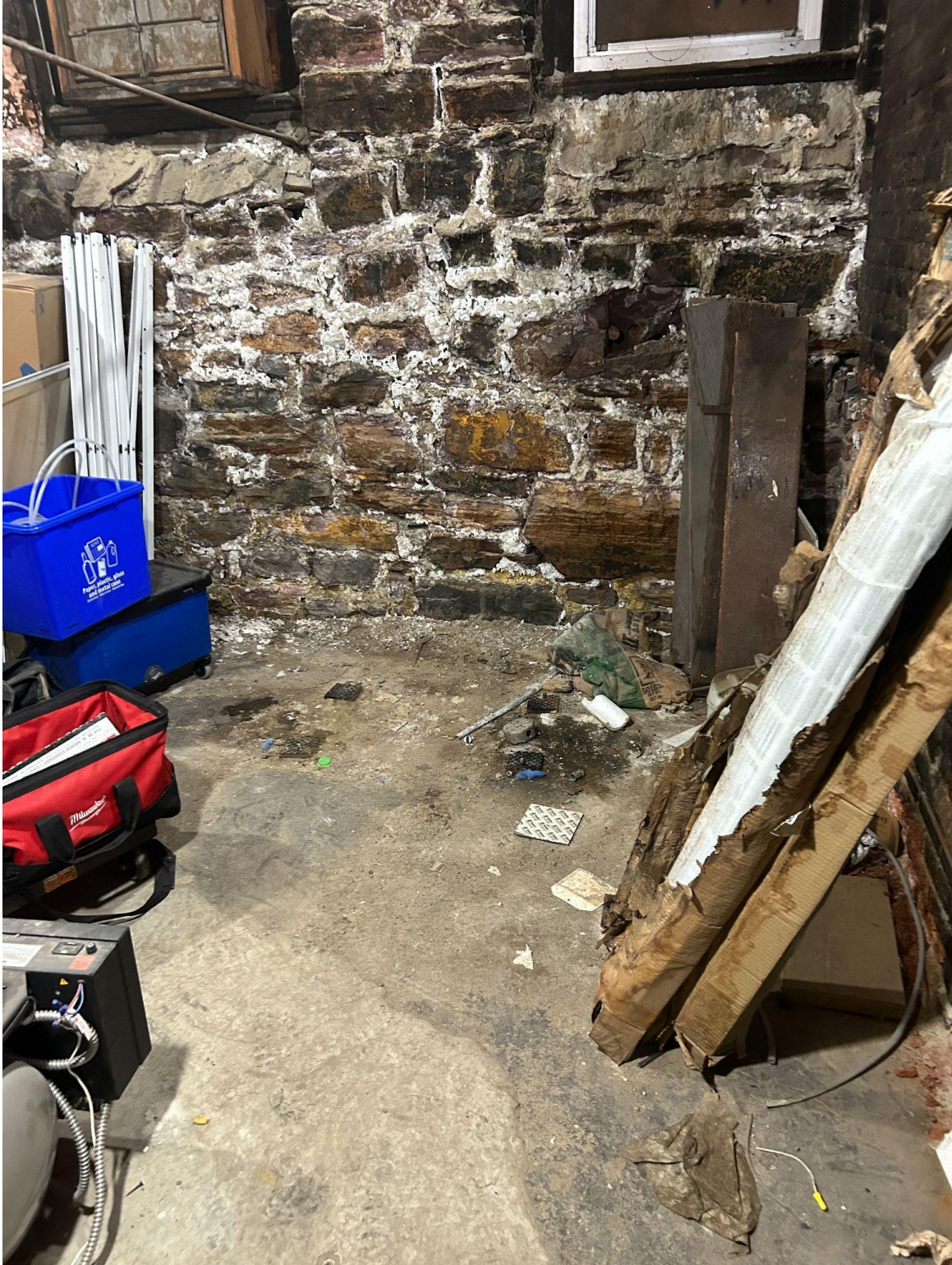
The Building's old temperature control air compressor was removed on Thursday (5/23), making way for the new electronic temperature controls that will be installed for the new Mechanical equipment and school upgrade.
