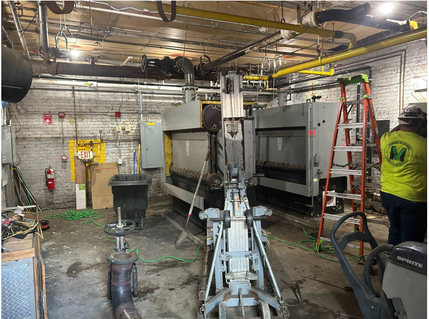
Beginning of the demolition of the Boiler Room.
