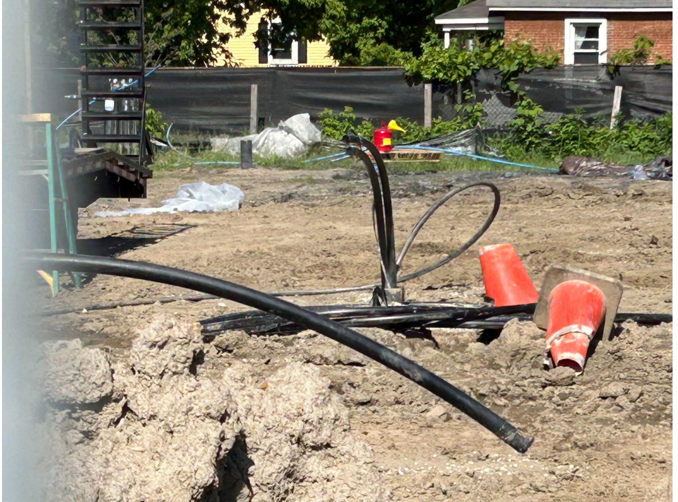
The process of grouting the wells.
