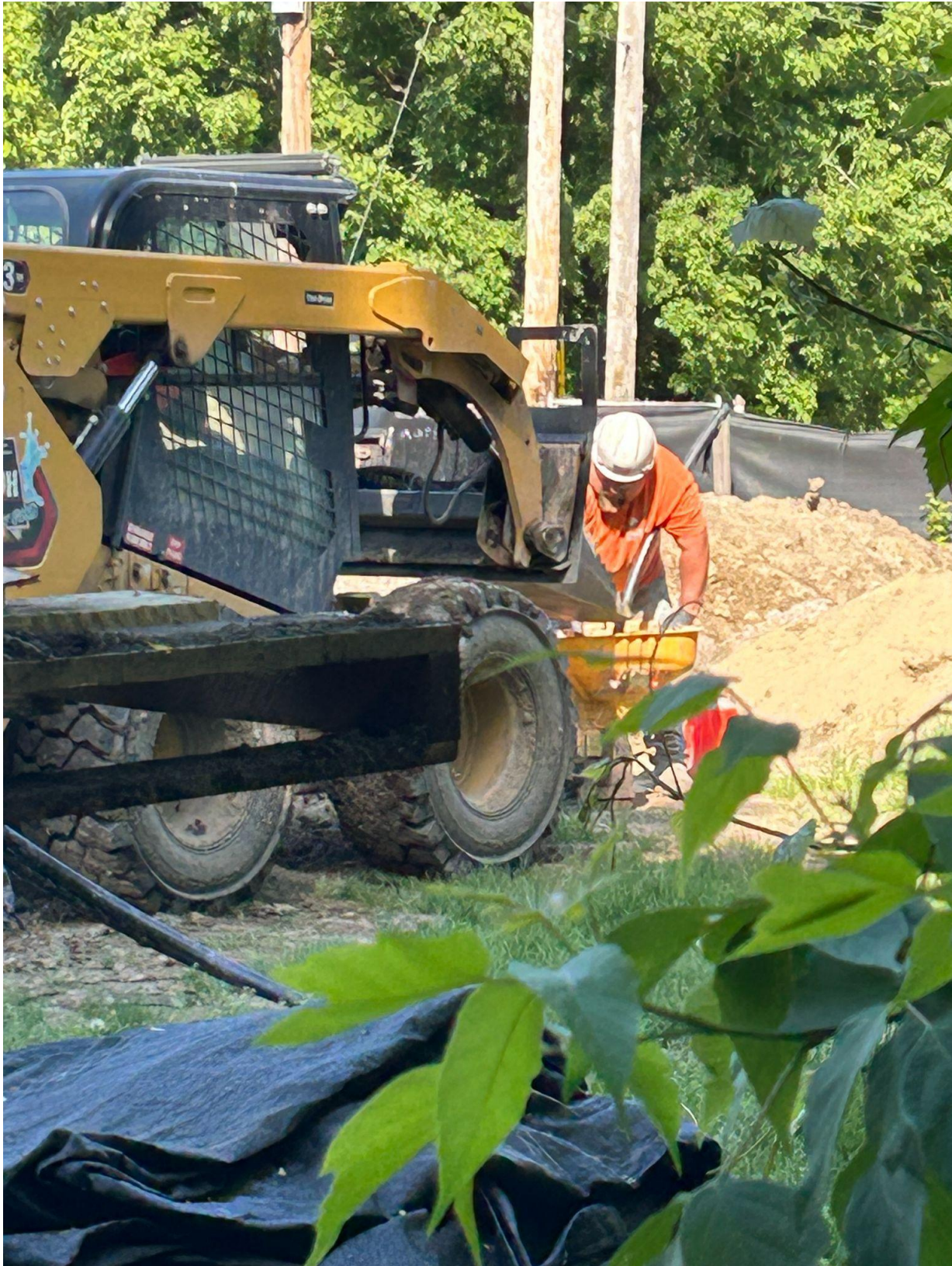
The process of starting to fill up the wells. Small gravel is placed within the well.
