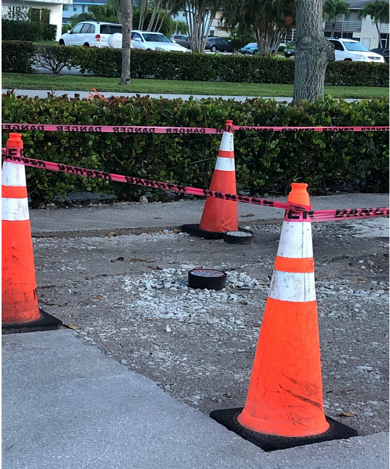
BERKSHIRE SECTION- SHUT OFF VALVE INSTALLATION COMPLETE. PAVEMENT WILL BE RESTORED THIS WEEK.
