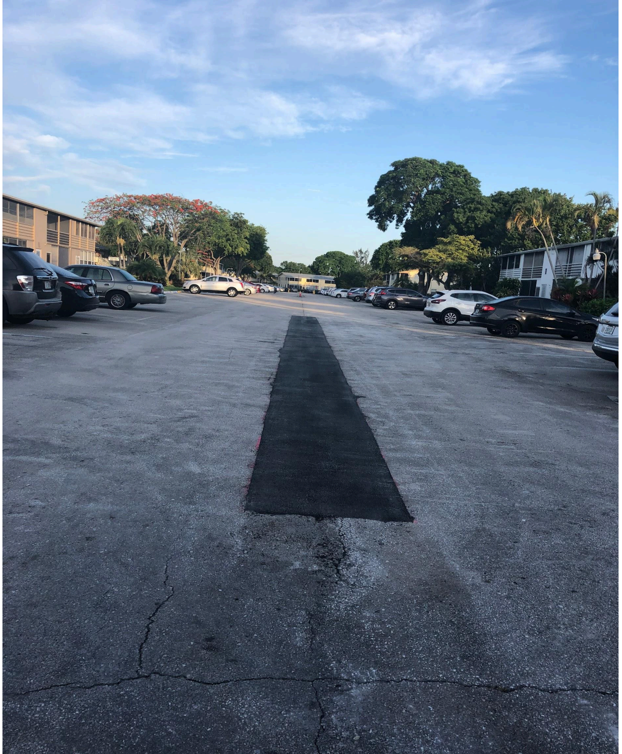
CAMDEN SECTION- PAVING REPAIR COMPLETE.
