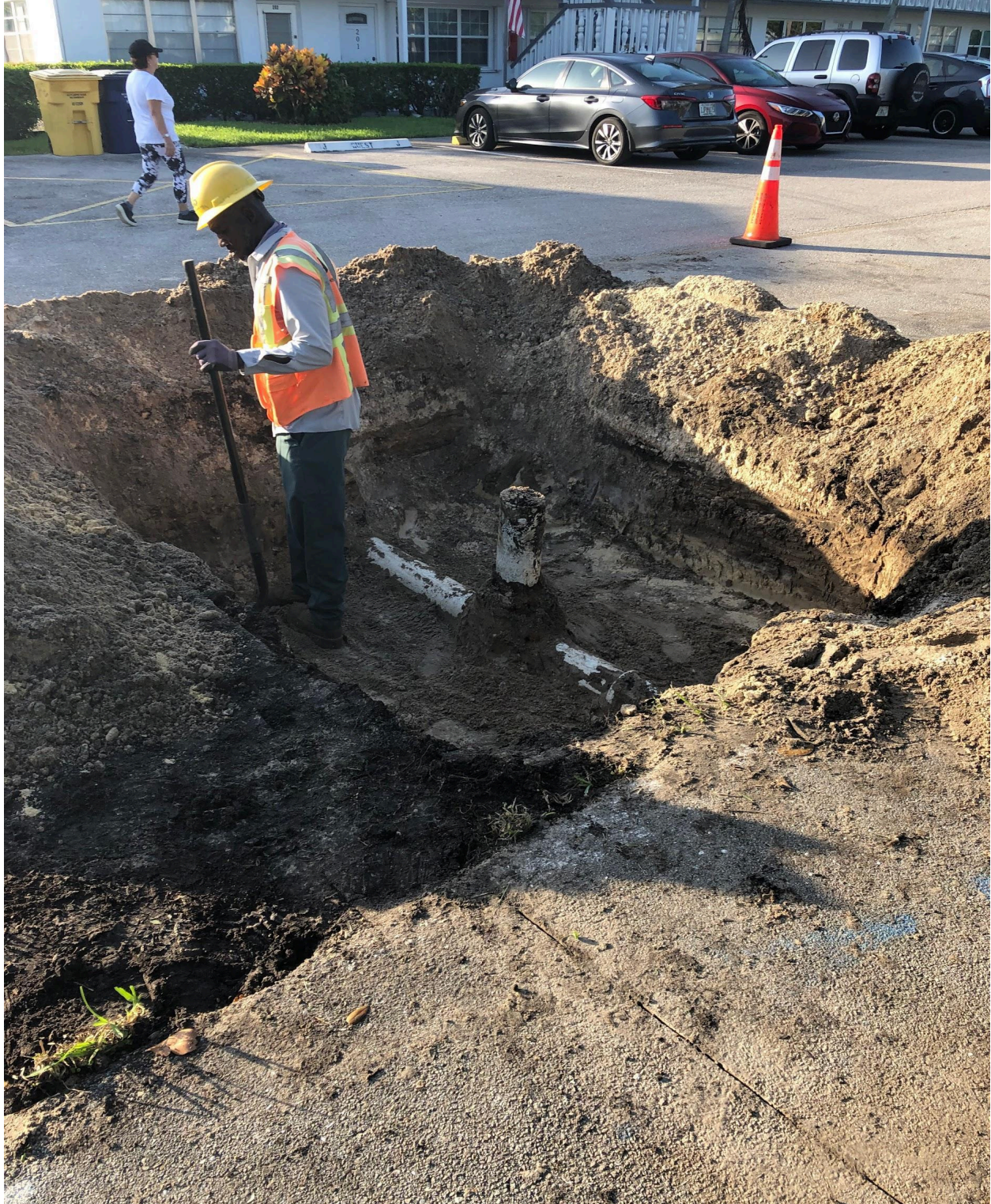
BERKSHIRE SECTION- A SHUT OFF VALVE HAS BEEN INSTALLED AT THE BRANCH LINE THAT CONNECTS THE MAIN WITH BERKSHIRE J AND K.
