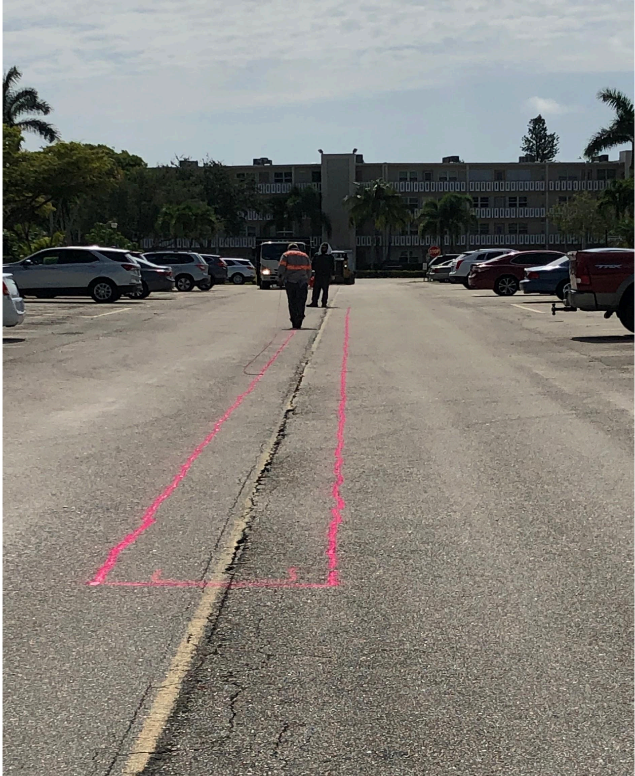
CAMDEN SECTION- ATLANTIC SOUTHERN PAVING MARKS OFF A DETERIORATED SECTION OF ROAD.
