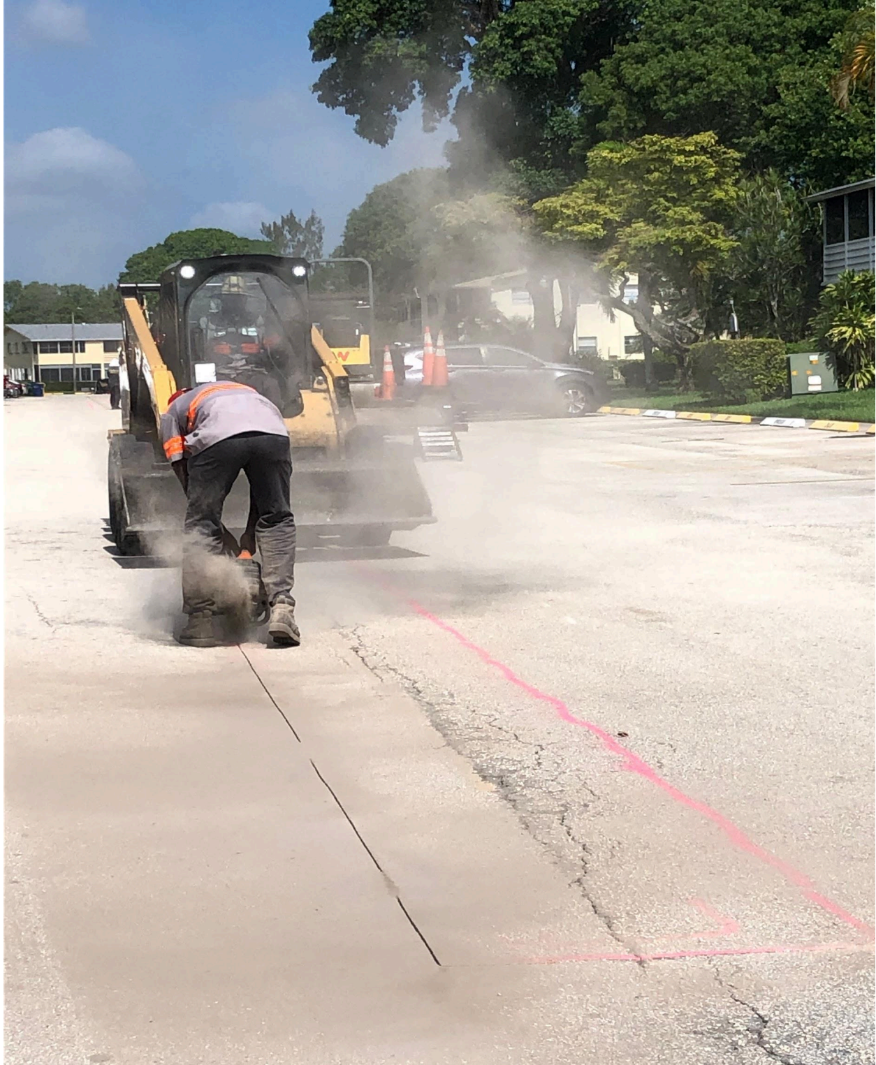
CAMDEN SECTION- A DETERIORATED SECTION OF ROAD IS SAW CUT AND REMOVED.
