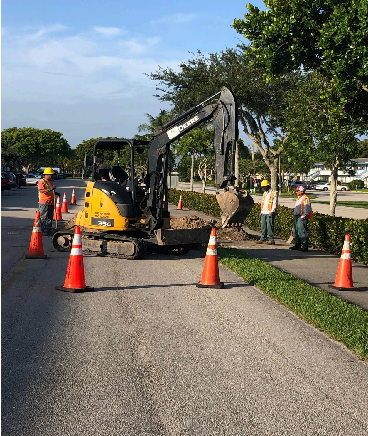
BERKSHIRE SECTION- J&D CONSTRUCTION EXCAVATED POTABLE WATER LINES LAST WEEK.
