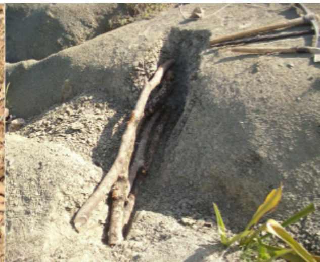
Picture 7: Reinforcement of trenches across
