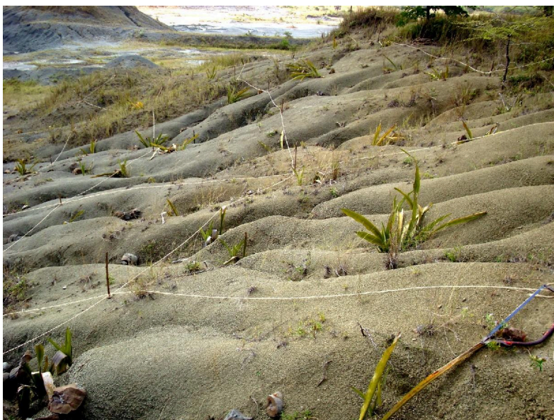
Picture 4: Preparing the excavations by marking with sisal twine
