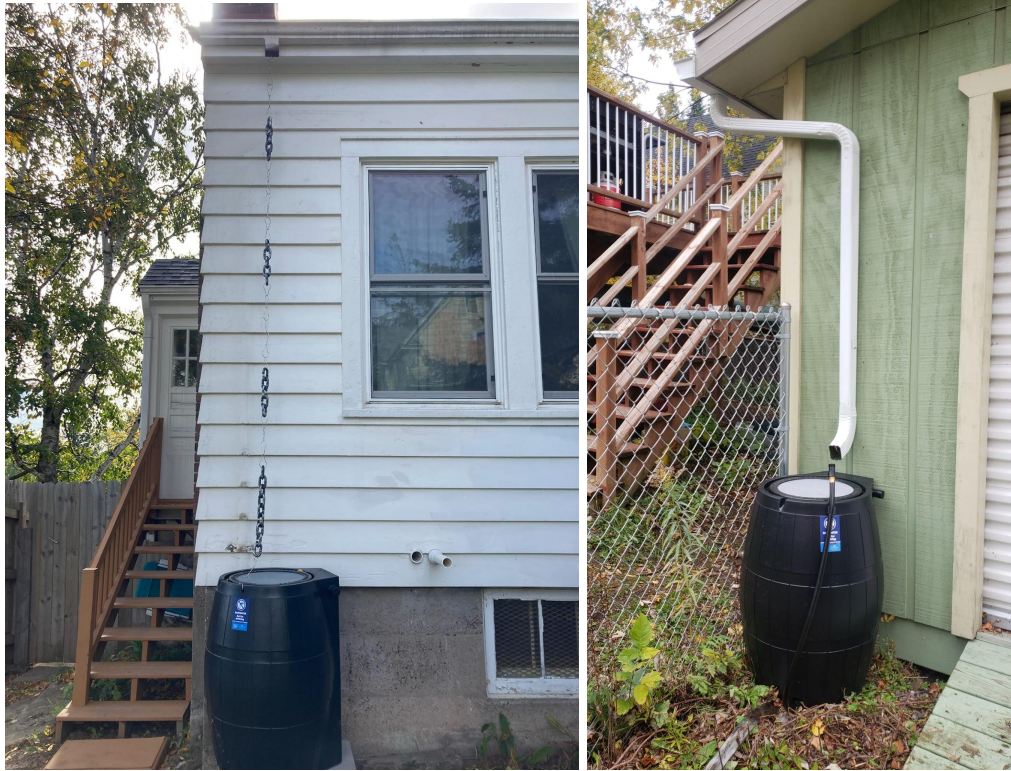
Image 7. Two rain barrels provided and installed. The rain barrel on the left was installed by the resident with a rain chain. Photo by L. White. The rain barrel on the right was installed by Community Action Duluth Community Construction along with a small length of gutter and downspout. Photo by Ron with Community Construction.
