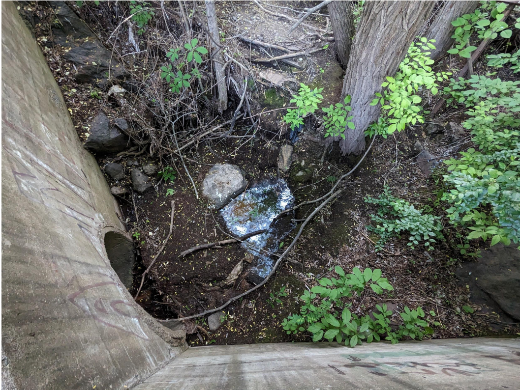
Image 5. Inlet culvert of 32nd Ave West Creek at Walbank Park in Lincoln Park; the creek runs entirely underground from this point onwards. Photo by M. Rodman.
