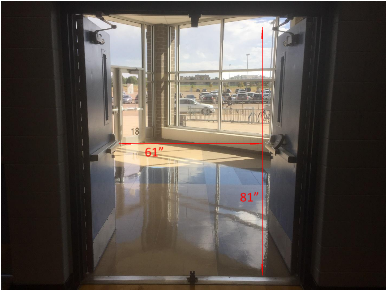
Door #5 – Performance Gym to Hallway
