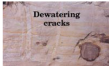
Dewatering cracks in Sandstone
