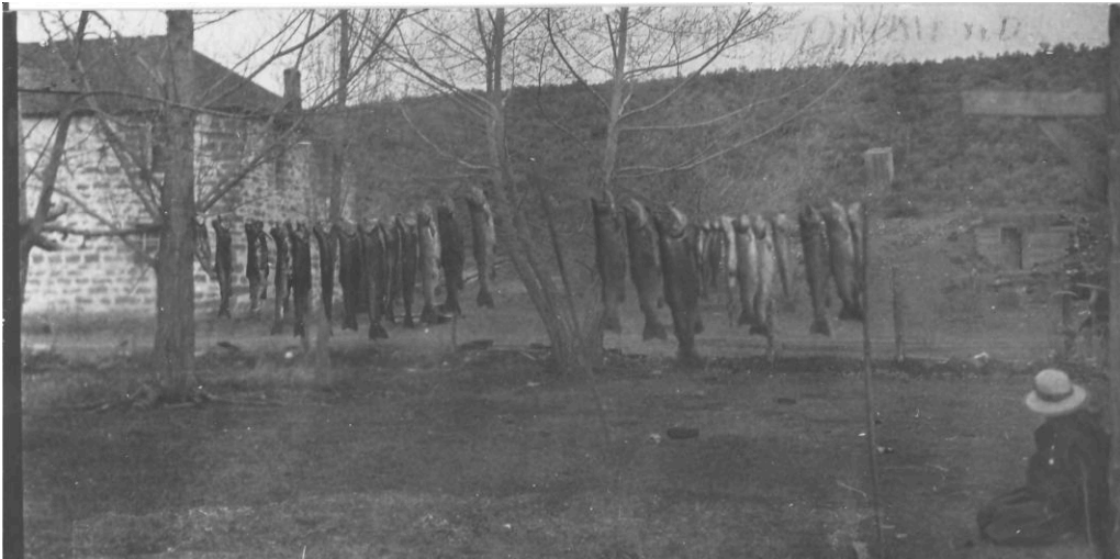
Figure 33. Historic photo taken in Diamond shows off a large catch (note this may be a mixed catch that includes redband, and also steelhead and Chinook salmon from the nearby South Fork of the Malheur River). (Credit: Claire McGill Luce Western History Room, Harney County Library).
