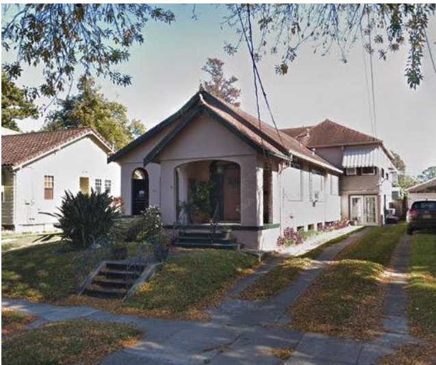
Photo: The Germann home at 4475 LaFaye Street in New Orleans, as seen by Google Street View in 2016. When the Germanns lived in this home it was the tiny modest shotgun house in front; the huge rear building and the stucco exterior were later additions.
