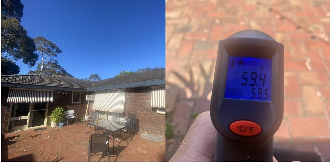
Figure 9: Ben's house gets minimal shade. The brick patio absorbs and retains the sun's heat, reaching up to 60°C.
