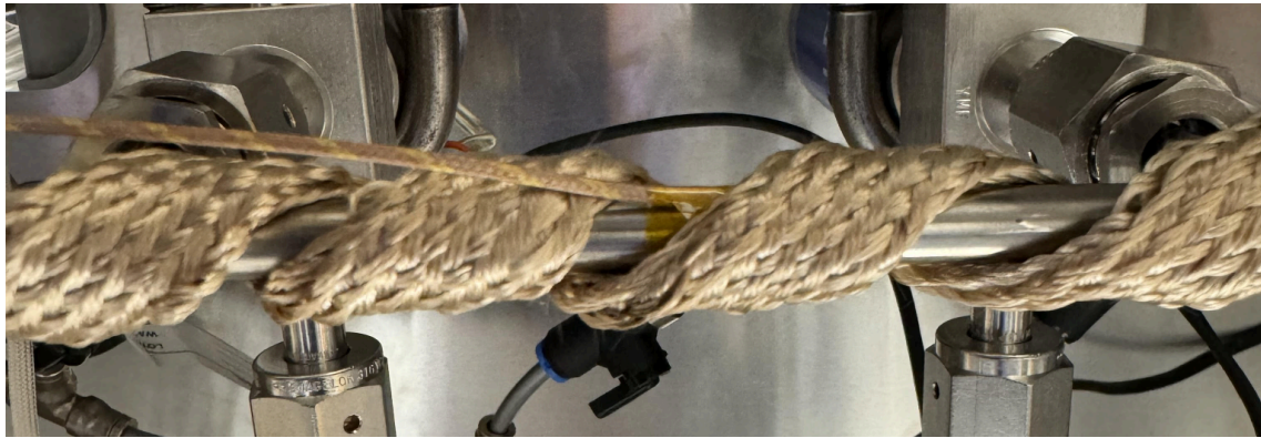
c. Example of properly mounted heating tape and thermocouple
