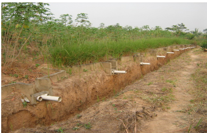
Plate 3: Trench dug down the 45 % slope for installation of sedimentation drums to receive runoff and soil loss passing through Usual Practice and vetiver grass buffer strips.
