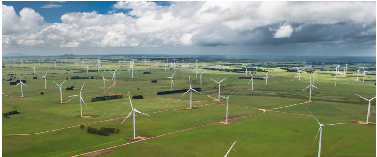
Figure 1: Capricorn Ridge Windfarm in Sterling County, Texas
