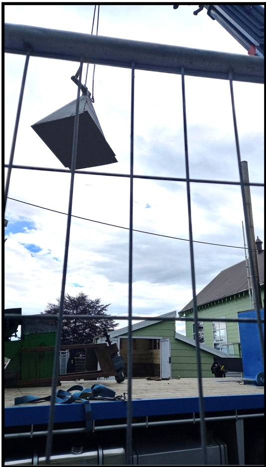
On the back of the truck the boiler and auger. Hanging on the end of the crane is the old coal hopper.
