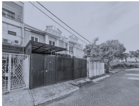
Figure 1. Existing Condition in the Citra 2 Housing, Jakarta Source: Field survey 2025
