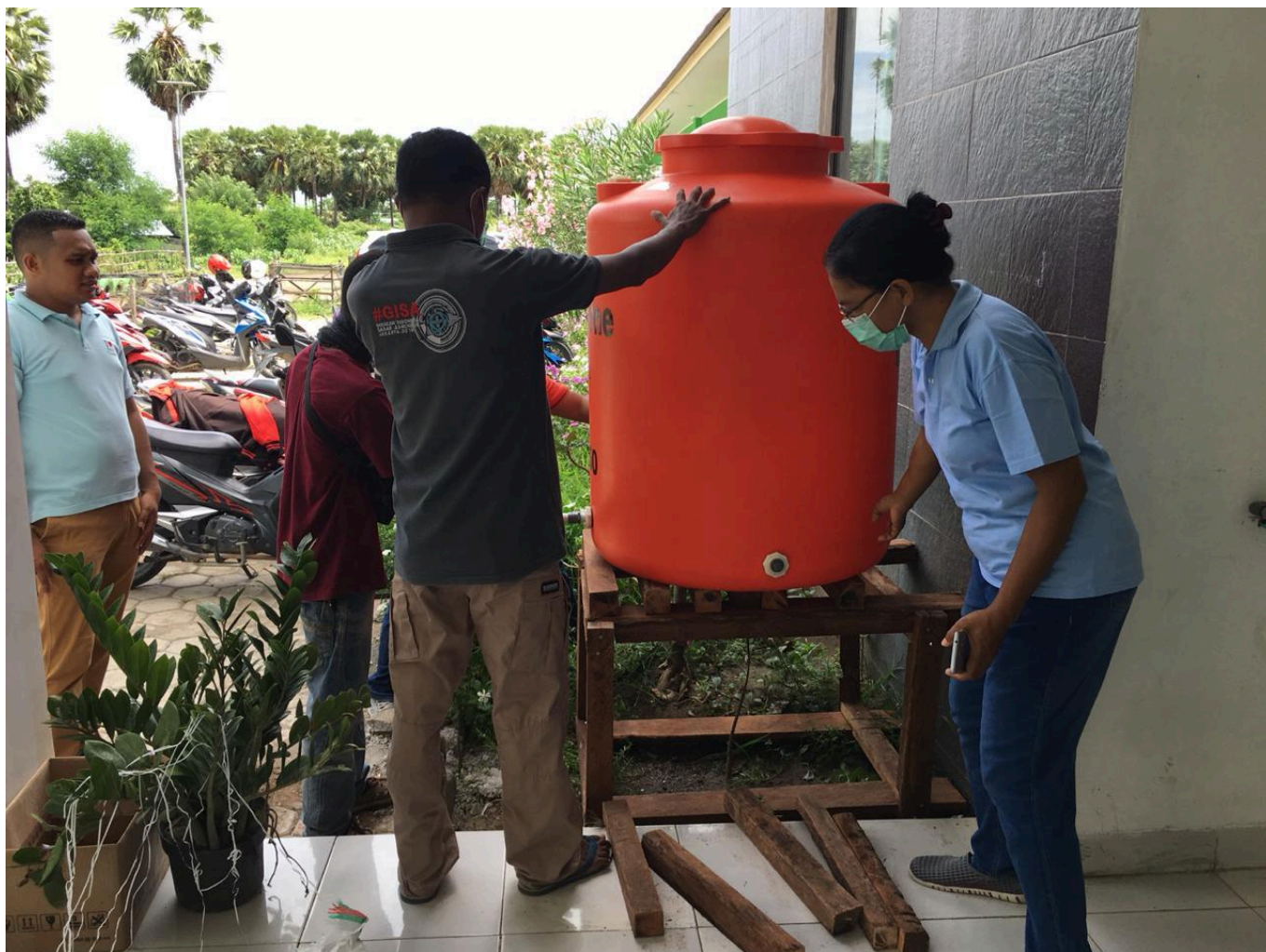
Figure 2 The installation of handwashing station in Aeramo Hospital
