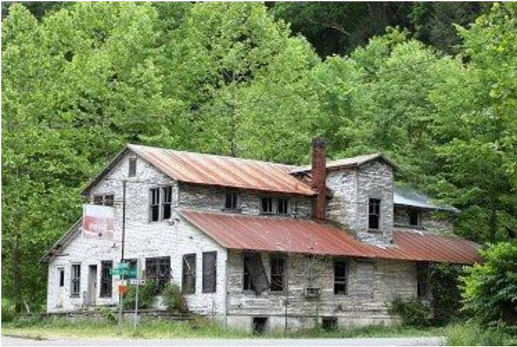
Former Virginia Banner Coal Corp. company store in Trammel, Dickenson County, Virginia. (Photo courtesy of Bluebird's Blog )
