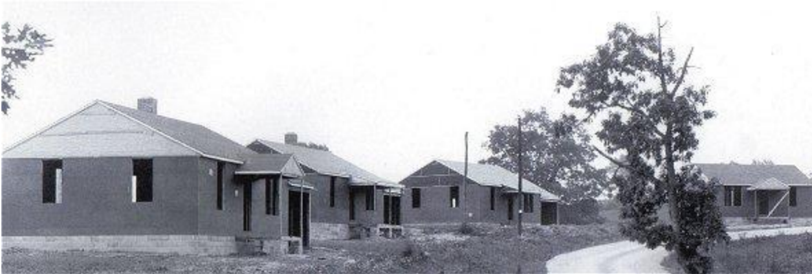
Photo of homes being constructed by Stonega Coal and Coke Company in Keeokee in 1946. (Image from Ed Wolfe's book "Coal Camps, Tipples, and Mines")
