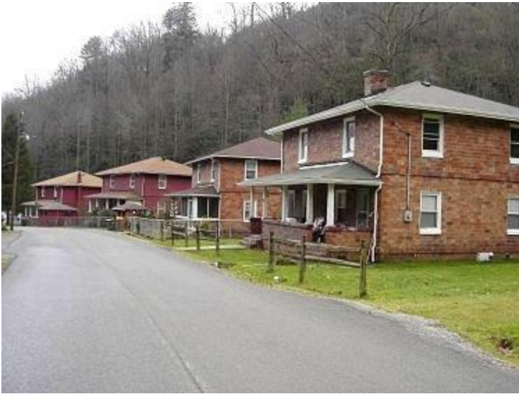
These red block company houses in Derby, VA represent the last coal town built by Stonega Coke and Coal (not counting their rebuild of Keokee in 1947). Derby was constructed in 1922- 23 and so named because the officials of the company stopped to tour their new town on the way to the Kentucky Derby. The "model" coal camp was added to the National Register of Historic Places in 2004. (Jan. 2007 image by author)
