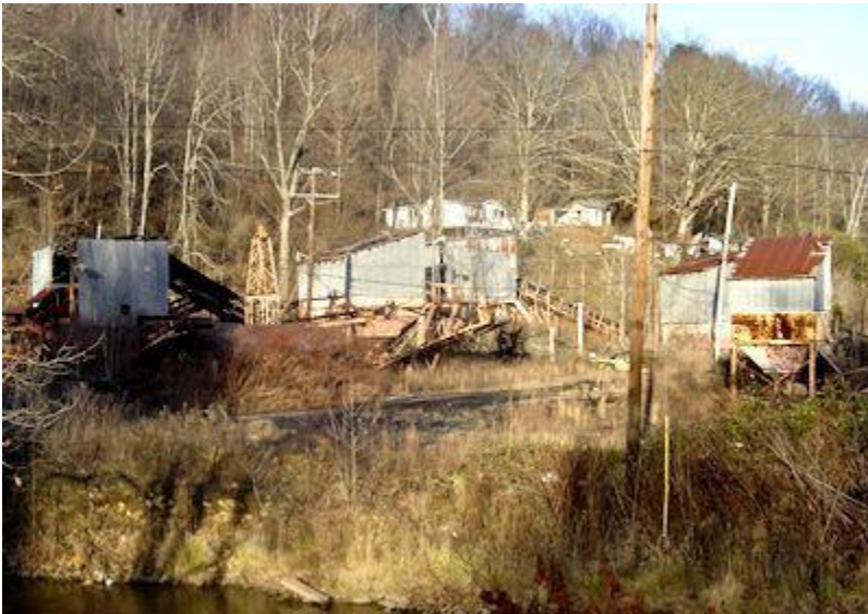
Idled coal loading facility near Pennington Gap, Virginia. (Dec. 2008 image by author)
