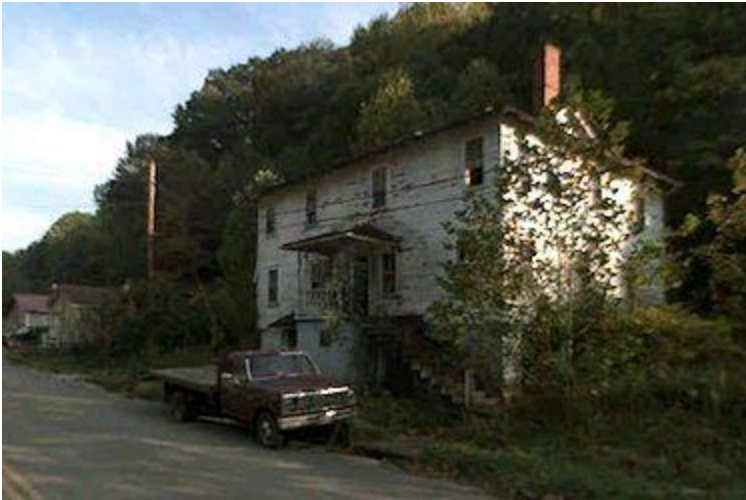
This larger structure at Trammel may have been the boarding house for single miners. (Image by others)
