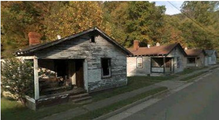
Former coal company houses still in existence at Trammel. (Image by others)
