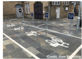
Marked non-standard cycle bays with mid-bar Sheffield stands (no tapping rails, poor contrast) Credit: Sam W. eling
