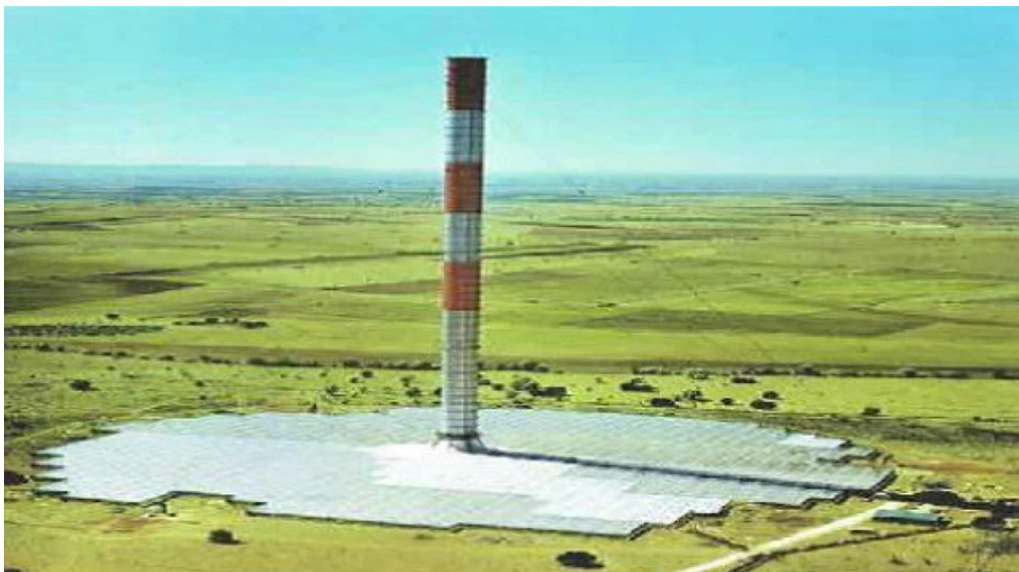
Figure 1-2: Solar chimney power plant in Manzanares.
