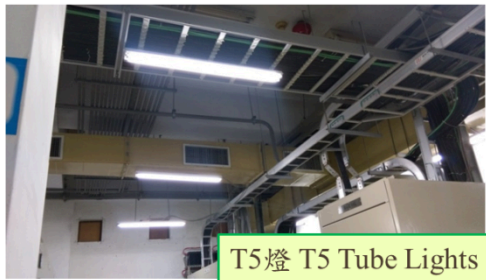
Energy Efficient Lighting fixtures
