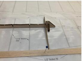
4. (2) R-1 ribs. Using the ROOT gauge, place R-1 at the proper angle on the spar. Add the second R-1 the same way, but align vertically. Add the rest of the R-2 ribs. Once satisfied with the fit, glue all the ribs in place to TE (note correct TE orientation) and spar.
