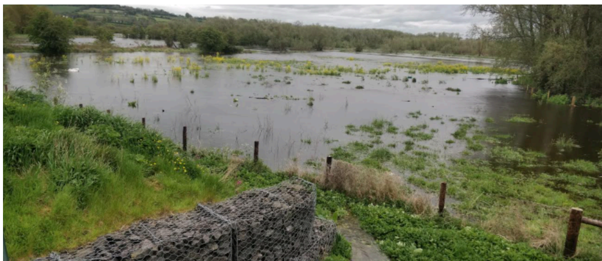
Figure 4. Flooding at Ecos Nature Park. Photo taken 21/05/2021. It is estimated the site stores 418,572tonnes of water in a flood of this size.
