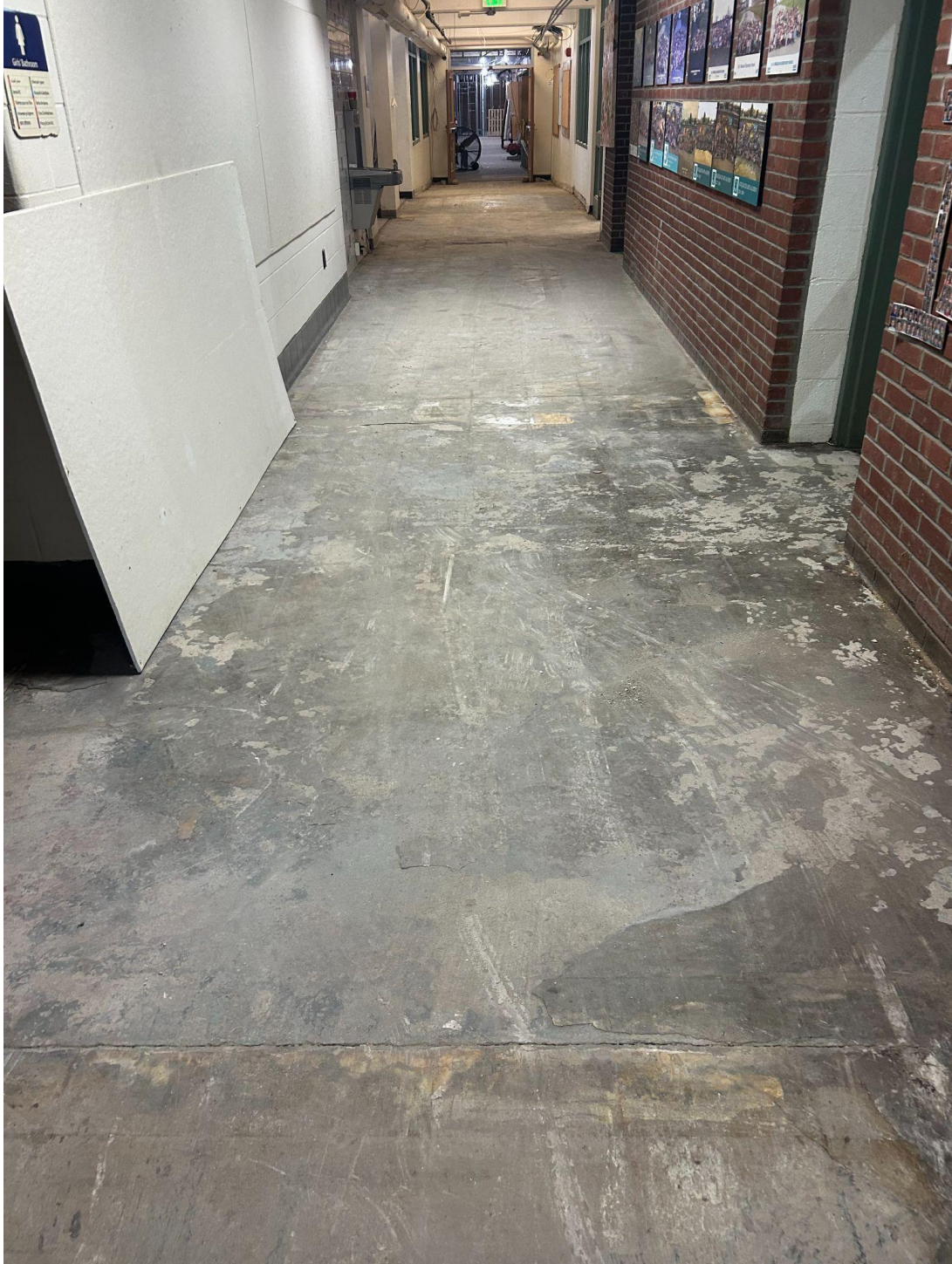
Picture showing the completely removed floor tile. This removal work in this corridor took the workers about an hour from start to finish, in removing the flooring tile.
