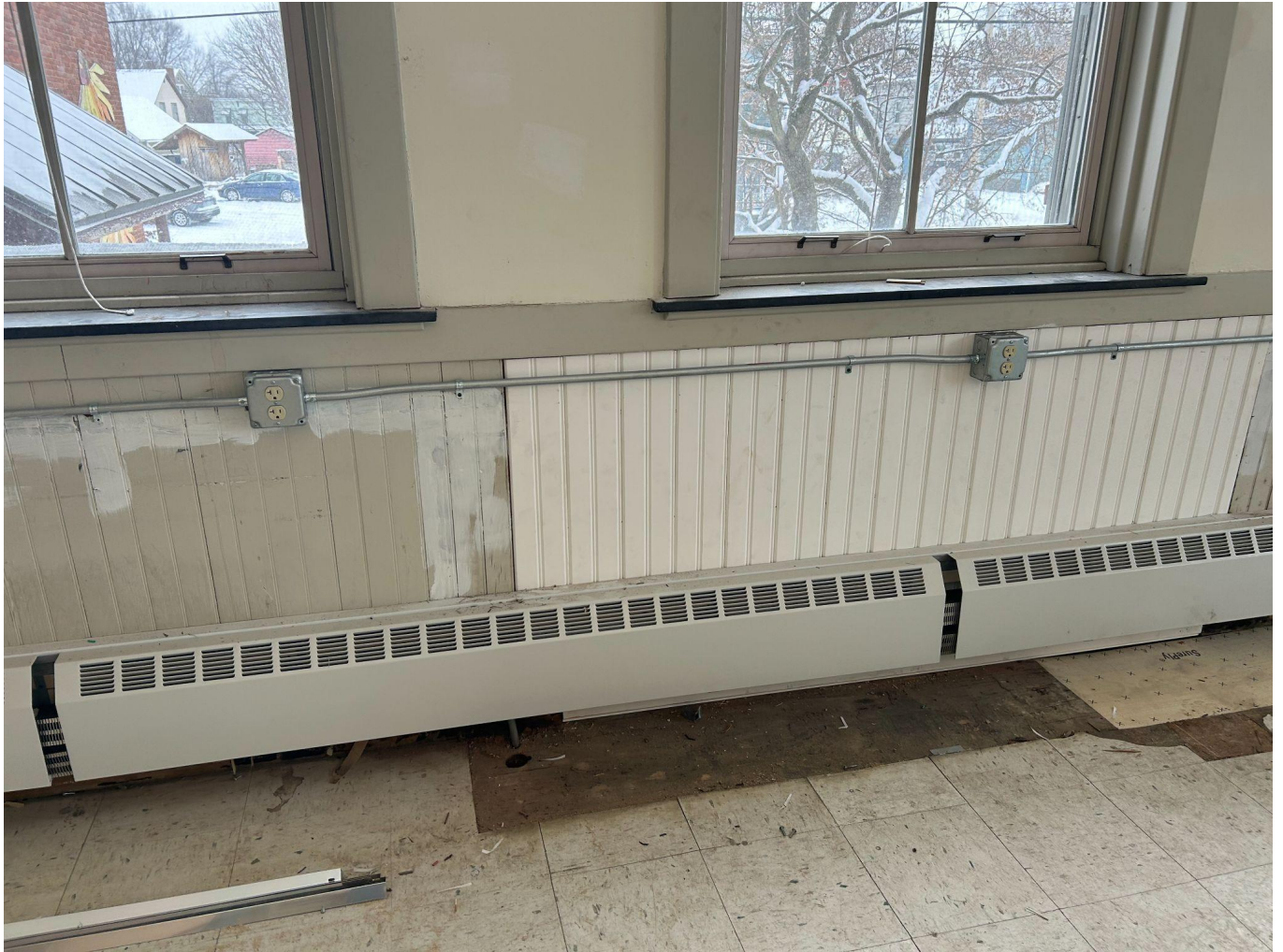
The BSD electrical team has finished placing the extra electrical outlets on the walls on the first floor in the 1904 wing of the building. They continue to chip away for the classrooms on the second floor.
