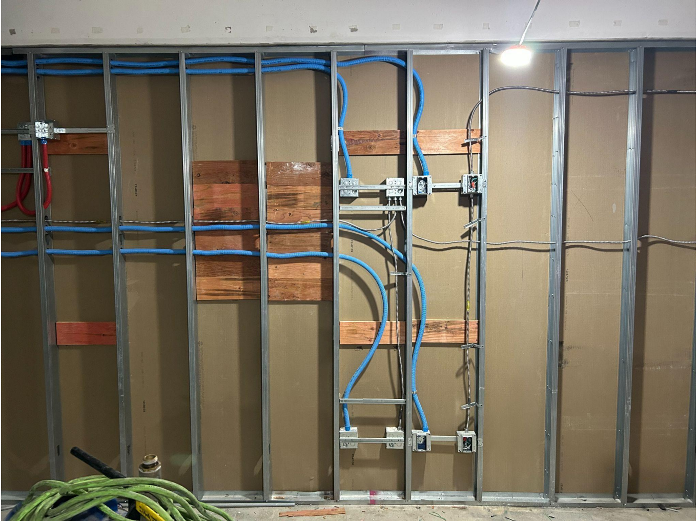
Blocking being installed in the walls of the classrooms in the 1965 wing of the building. Once the blocking is complete, sheetrock will be hung on this side of the wall, enclosing the blocking within the wall.
