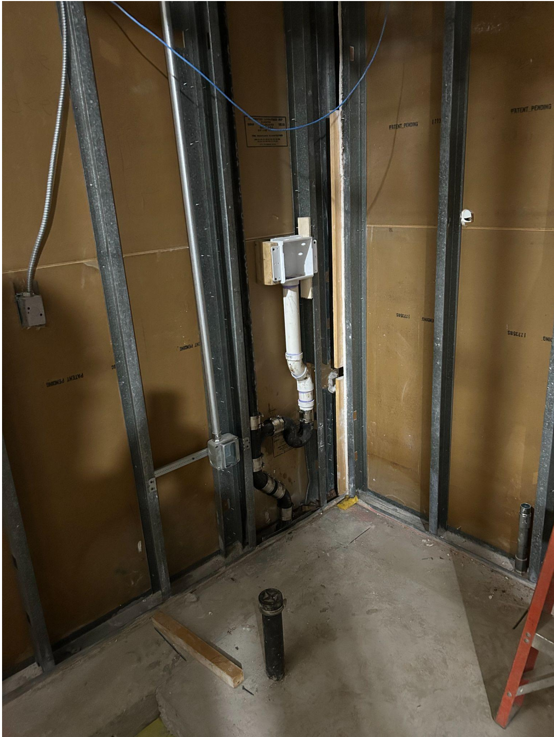
The plumbing contractors have finished roughing-in for the washing machine in the new Laundry Room that will be located in the 1965 wing of the building.
