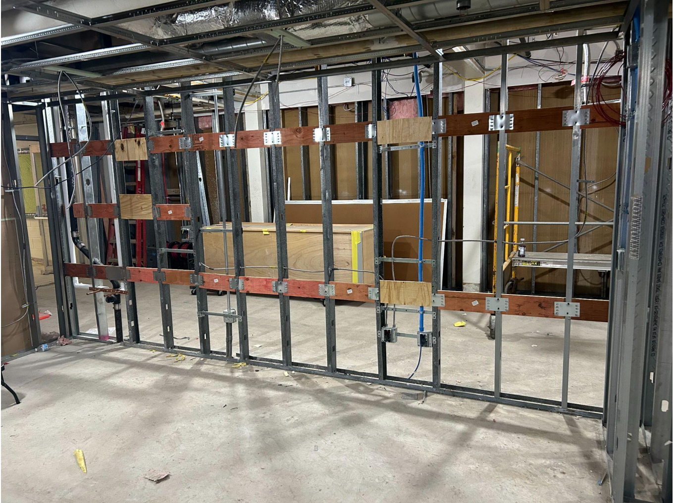
Another picture showing blocking being installed in the walls of the classrooms in the 1965 wing of the building.
