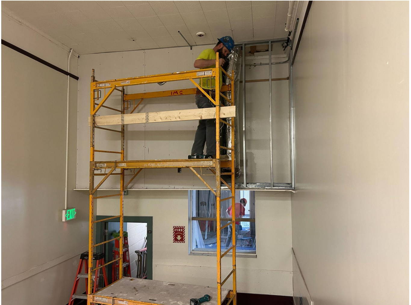
Soffits are being created to conceal the new ductwork needed for the ventilation of the rooms in the 1904 wing of the building.
