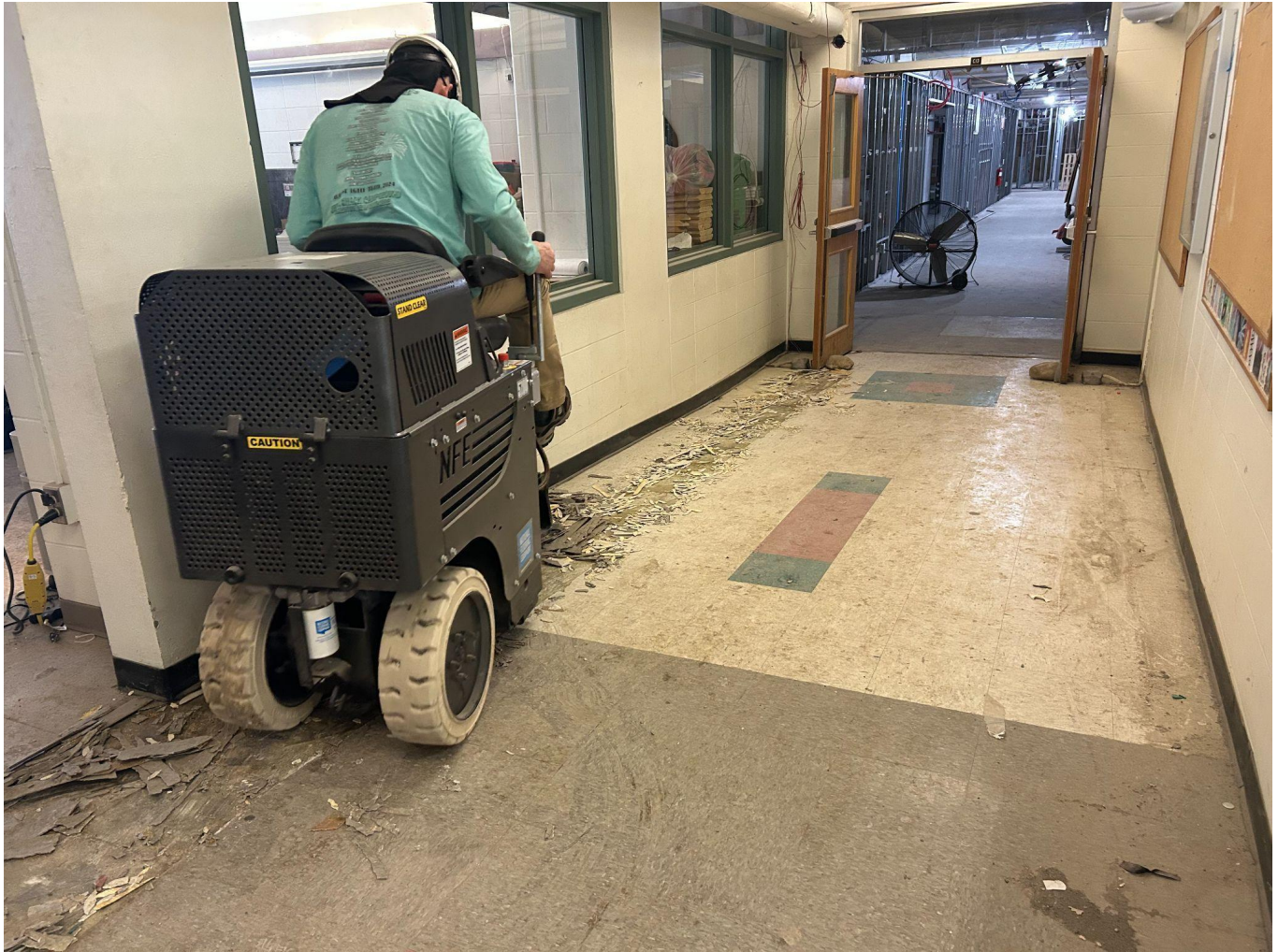
Picture showing a worker from Elegant Flooring on how they remove the old linoleum flooring. New flooring is slated to be installed throughout the building. This machine makes quick work of removing the glued down floor tile.
