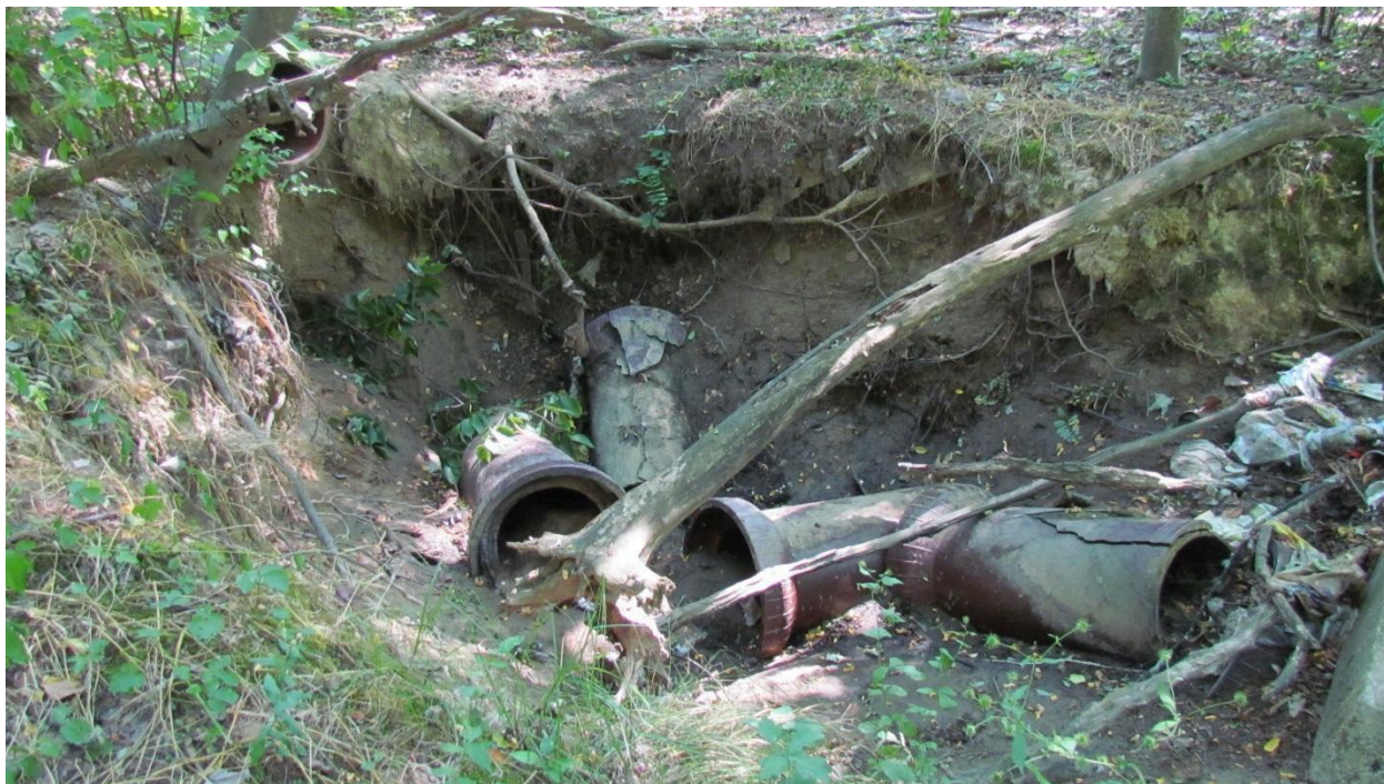
S4-23: Broken Drainpipe
