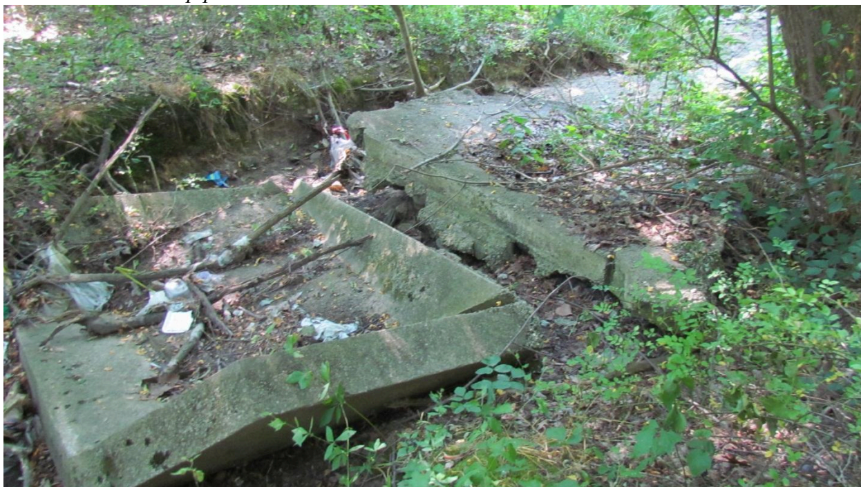
S4-23: Broken Drainpipe
