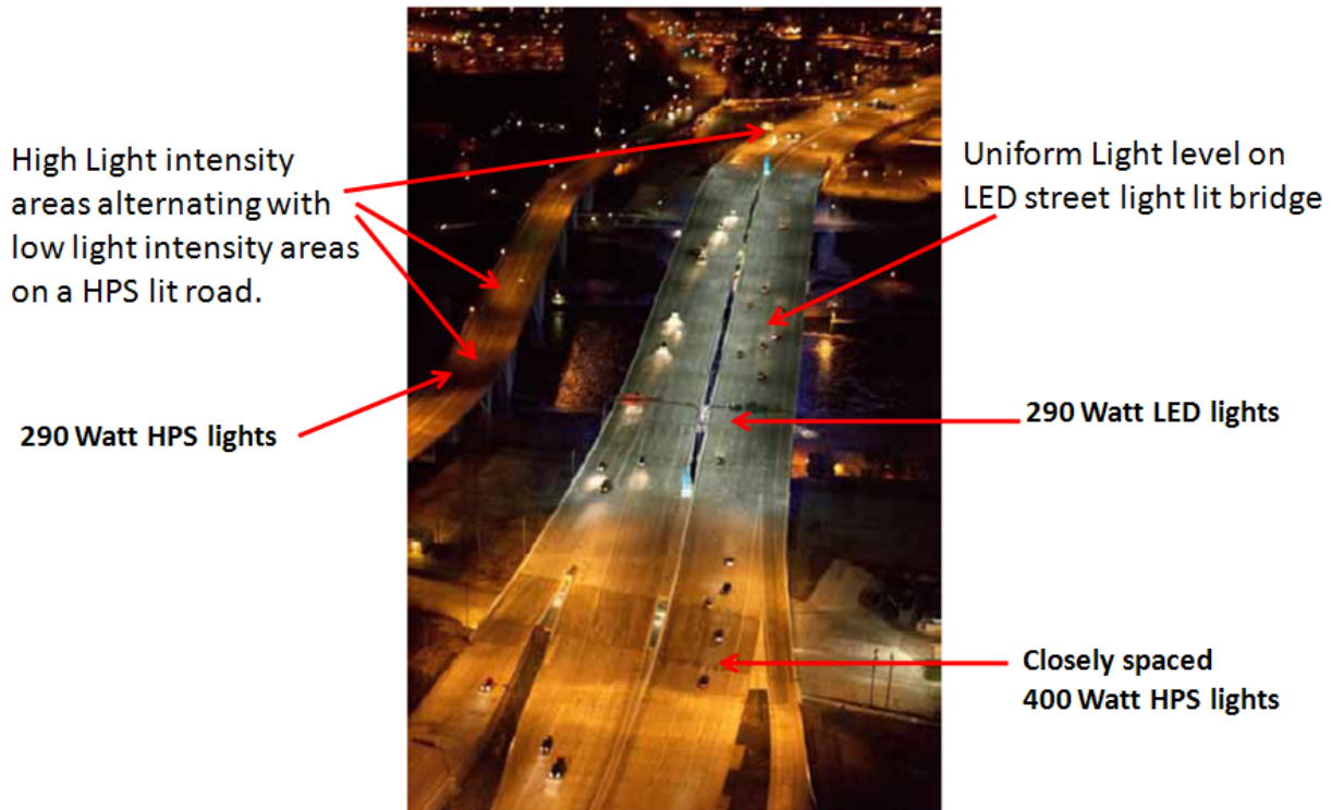
LED outdoor light project – I-35W bridge, Minneapolis
