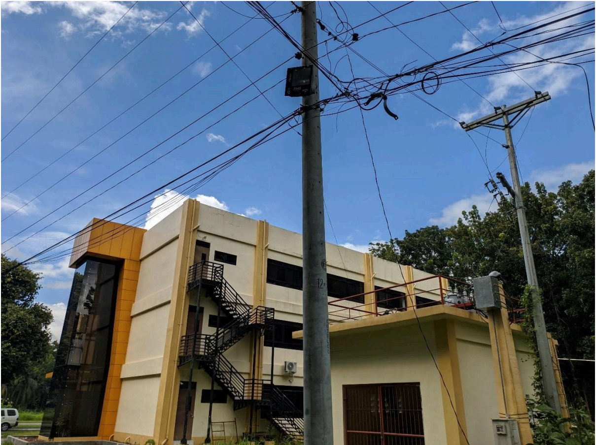
DOST BUILDING - EMERGENCY POWER GENERATOR
