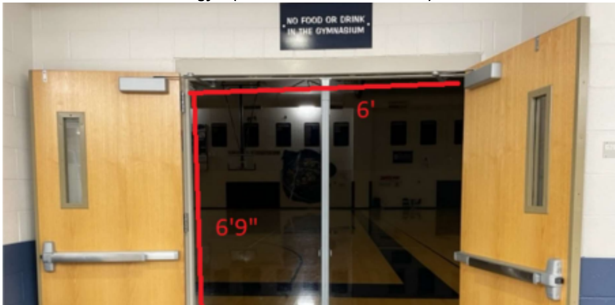
Unit exit from Performance gym (Middle bar will be removed)
