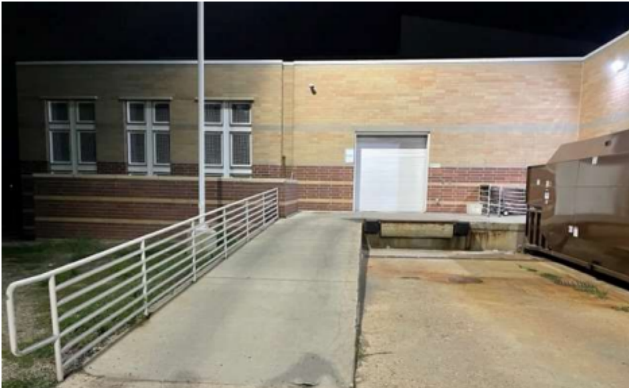
Outside Picture of prop door and ramp
