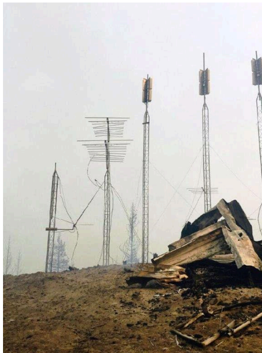
The Slide Ridge repeater site on August 27, 2015 (Courtesy of Ken Rau, K7YR)
