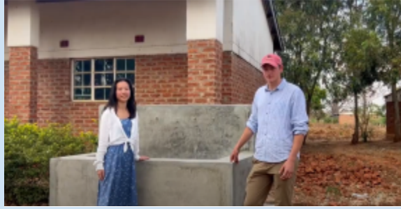
EWB with tap stands and sinks
