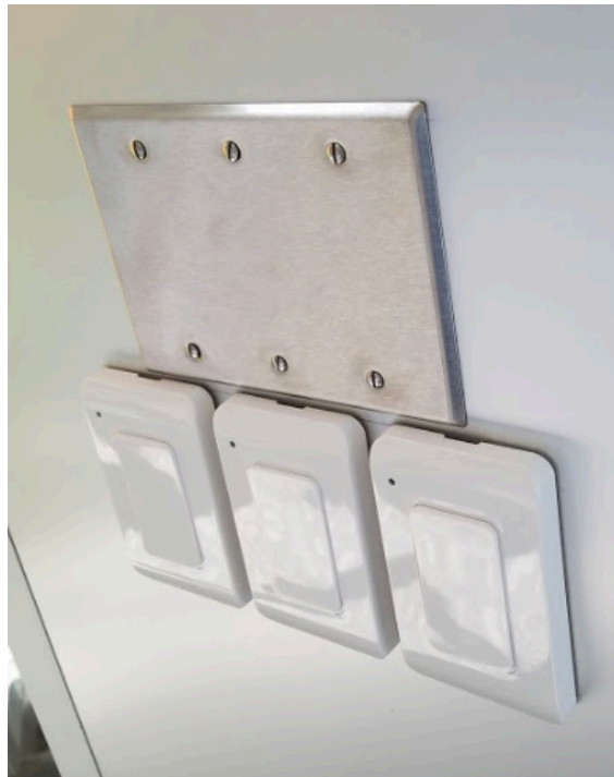
Wireless light switches below the old switch plate
