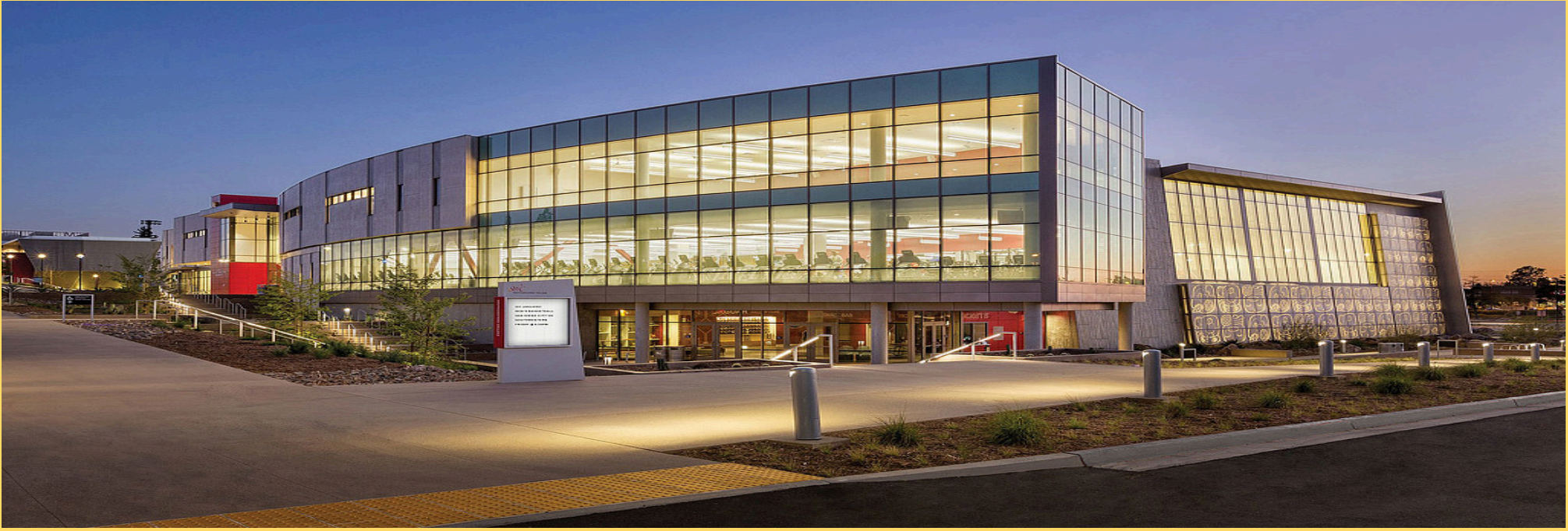
Picture Below: Gymnasium Front Entrance
