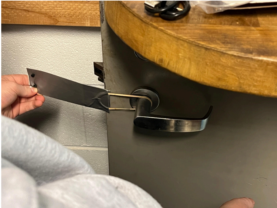
Figure 31: The rubber band keeps the door open
