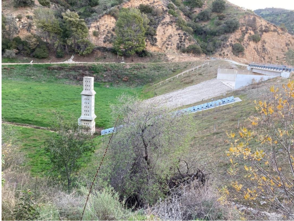
Figure 7: Little Dalton Debris Dam at delta of Little Dalton Canyon. Glendora Mountain Road is seen at the other end of the canyon. Photo taken Dec. 24, 2022.
