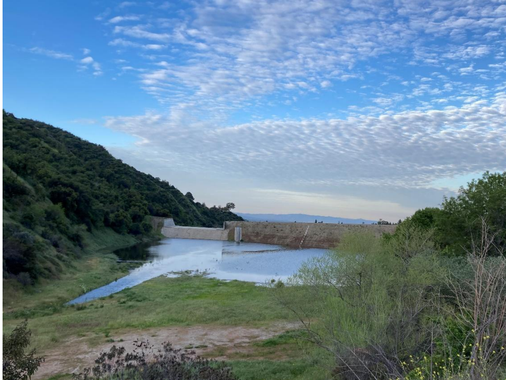
Figure 16, Big Dalton Debris Dam and Basin. The basin is only filled with water in wet years. Photo taken April 7, 2023.
