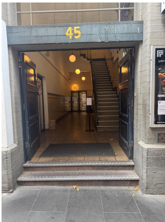
Picture 1: Steps from front path
