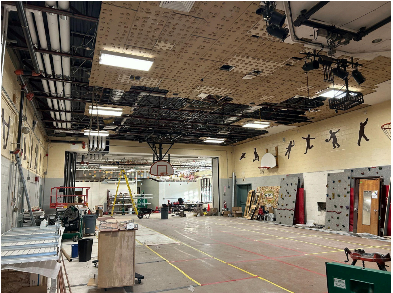
A picture showing the progression of the work going on in removing the old ceiling in the GYM.
