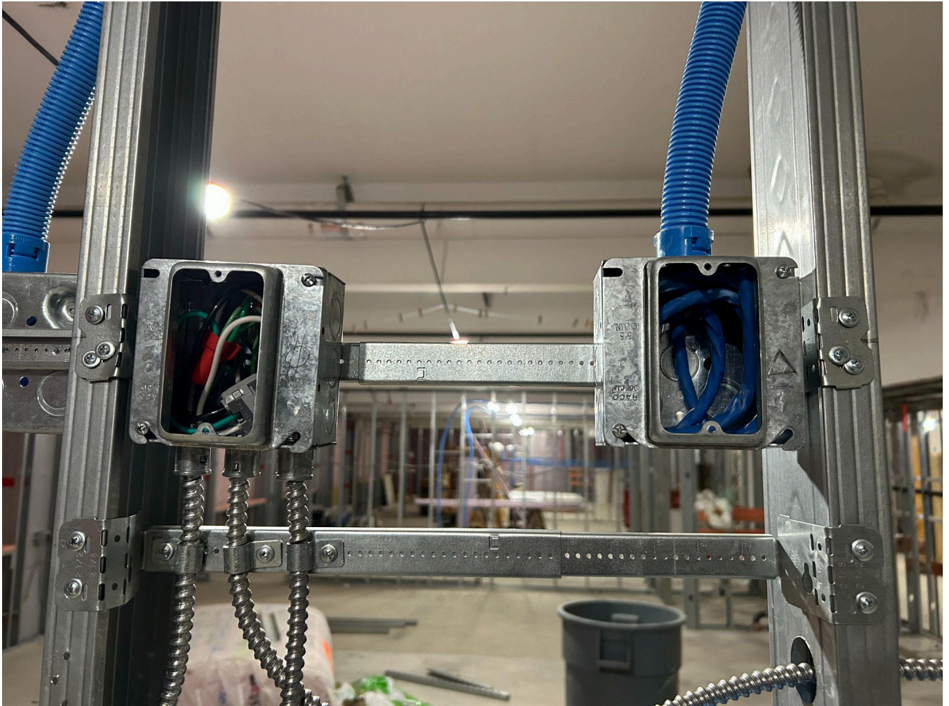
A picture showing the installation of wiring within the metal Jboxes for either the electrical outlet (Jbox on the left) or the data wiring (Jbox on the right) in the classrooms in the 1965 wing of the building.
