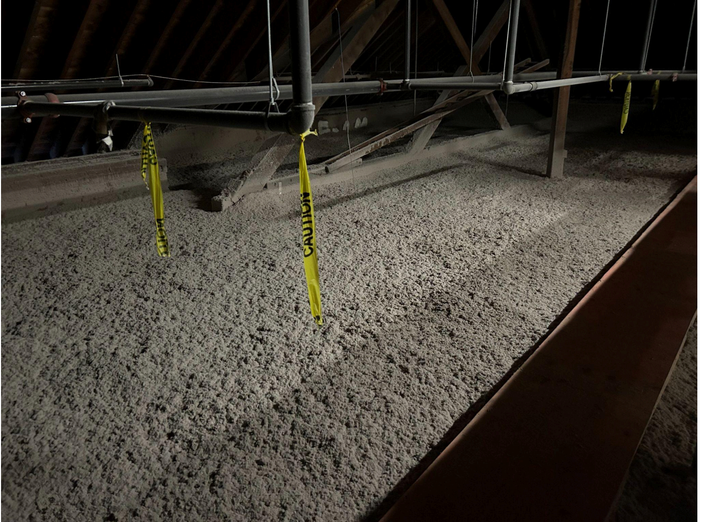
A picture showing the new insulation that has been installed in the Attic. This insulation covers the floor of the Attic.
