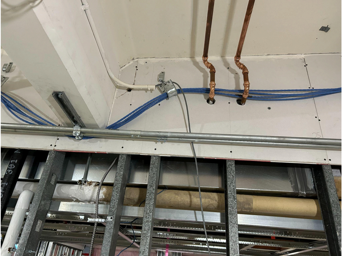
Picture showing the data wiring being hung on the corridor walls that will then be above the new ceilings.
