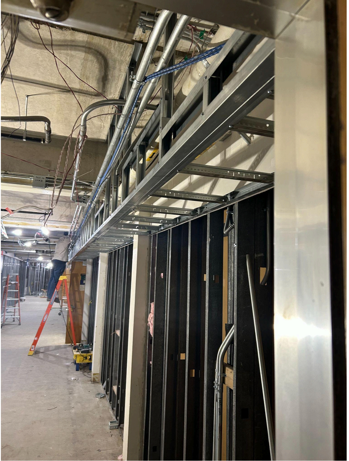
A picture showing the installation of the framing for the soffit in the corridor in the 1965 wing of the building.
