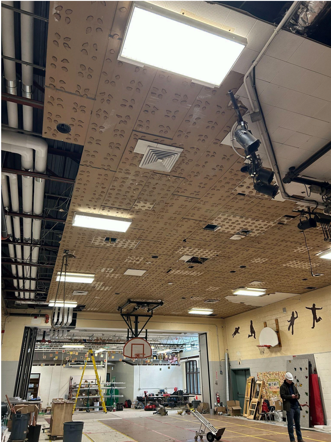
A picture of the GYM ceiling that is starting to be taken down. The GYM will have a new ceiling when construction is complete.
