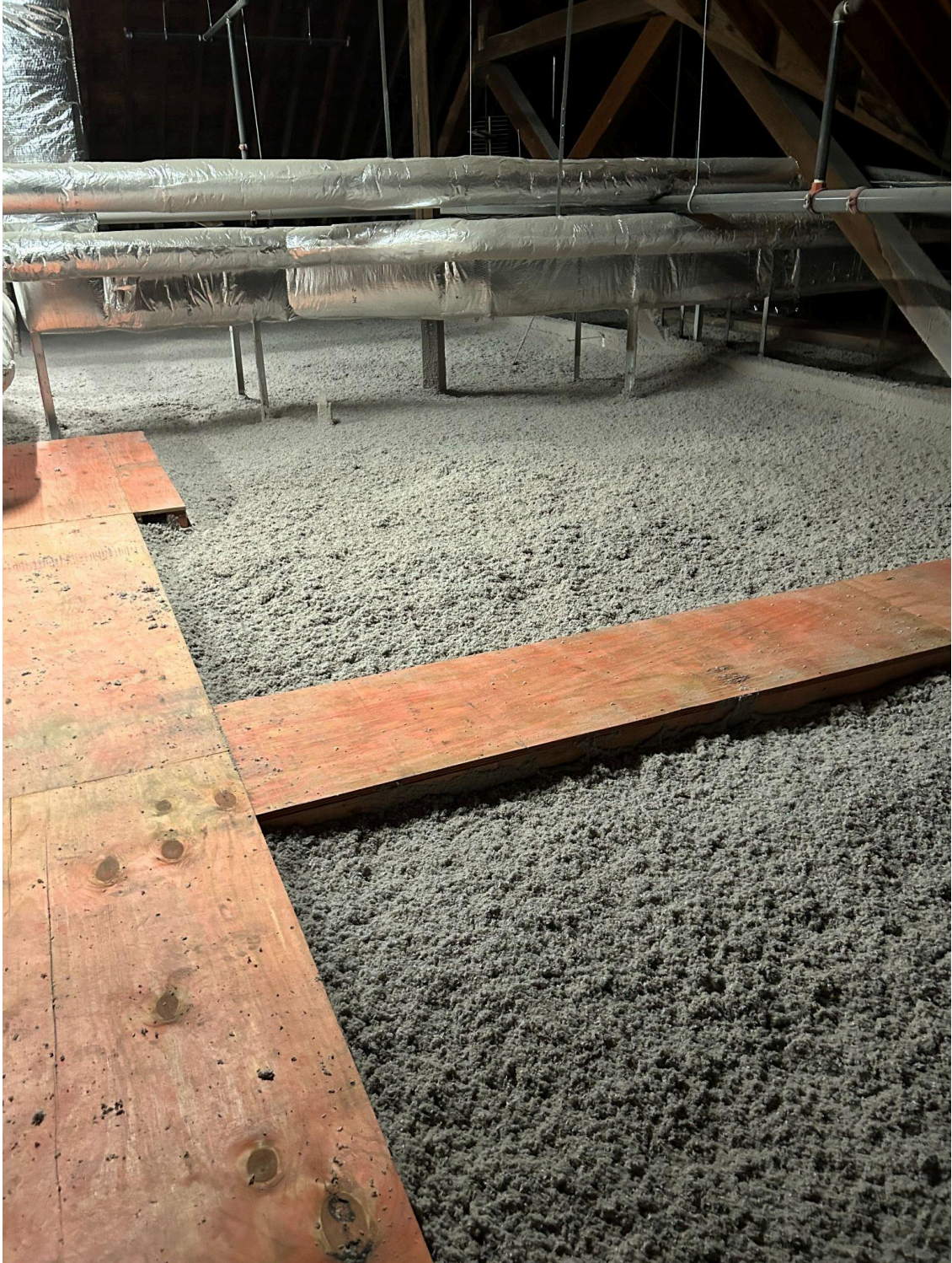
Another picture of the insulation in the Attic. A few weeks ago, we showed pictures of these catwalks being installed. The catwalks are now above the insulation and it is easier to walk around up in the Attic of the 1904 wing in the building.
