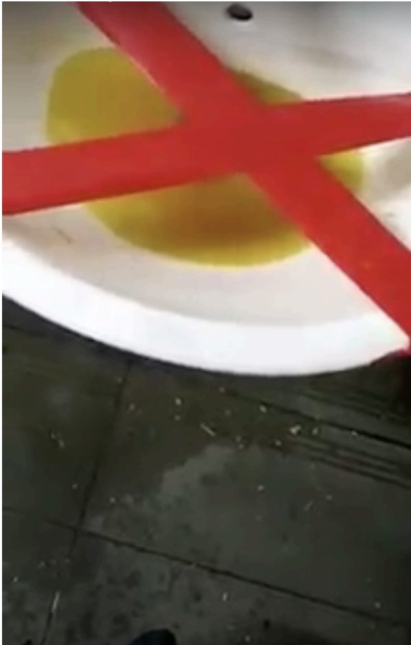
Figure 22: Faulty clogged and dirty sink
