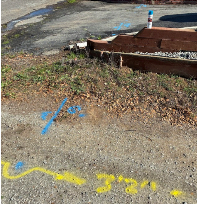
6' under the secondary driveway on the left side... on the right side the signal disappeared at 7' deep....
