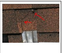
2. Use a pry bar to loosen the shingle where the flashing will be installed.
