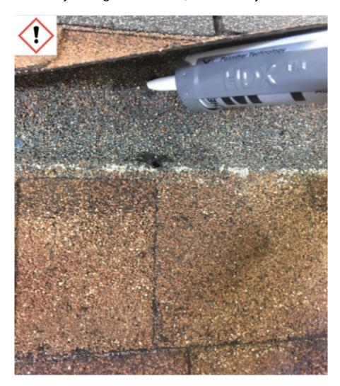
**IMPORTANT:** If any nails were removed due to the flashing card being in a highly visible location the nail holes <u>MUST BE SEALED!</u>
