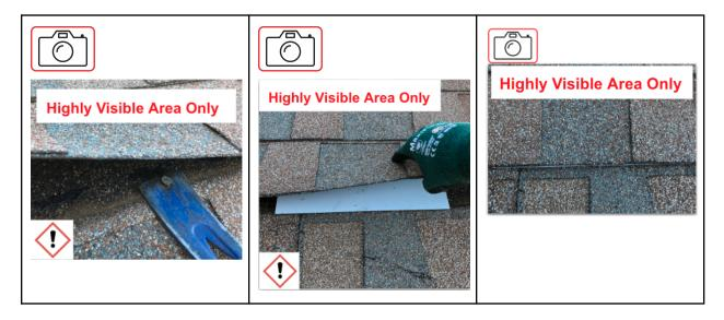
Anchor holes may require up to 3 card flashings, depending on where the holes line up with the comp layers. Ensure that all unused pilot holes have a flashing underneath them.
