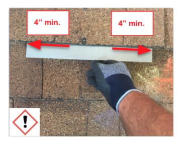
Butt flashing to the nails in the course above.
