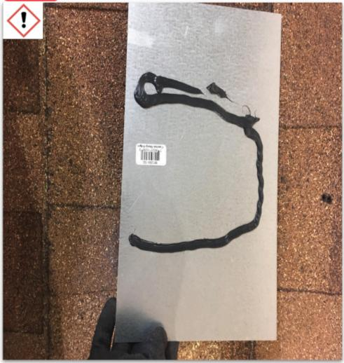
**IMPORTANT:** DO NOT CUT THE FLASHING. Flashing must be installed in the landscape orientation.
