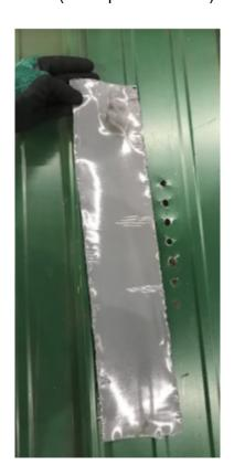
• Remove the backing and adhere the repair tape to the roof surface by laying down one end of the repair tape, working it in one direction and pressing out air pockets as you lay it down.
