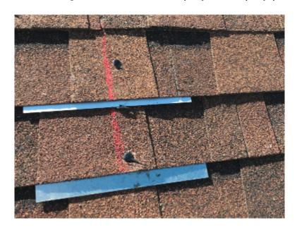
**IMPORTANT:** Once complete, any excess sealant above what is pictured shall be cleaned off of the roof surface.
