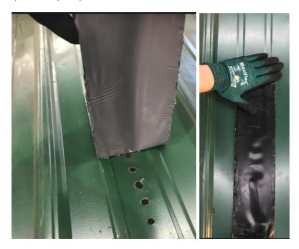
• Using the hand seam roller, apply firm pressure to the entire tape patch.
