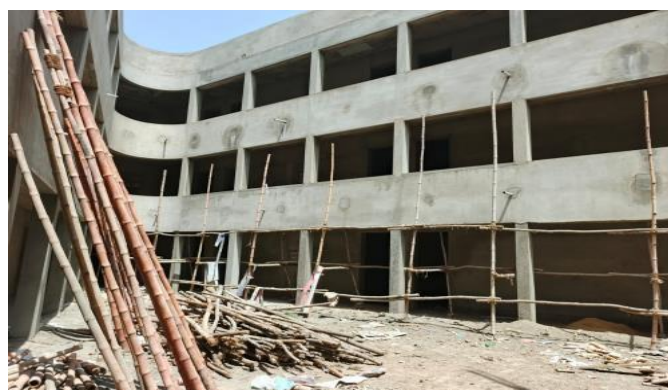
ITC Mega Building — construction progress
