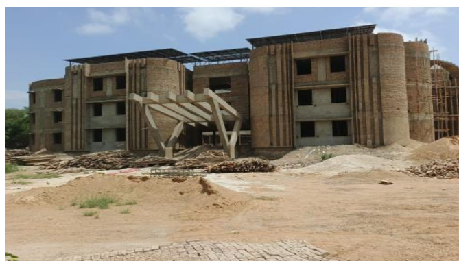
ITC Mega Building — construction progress
