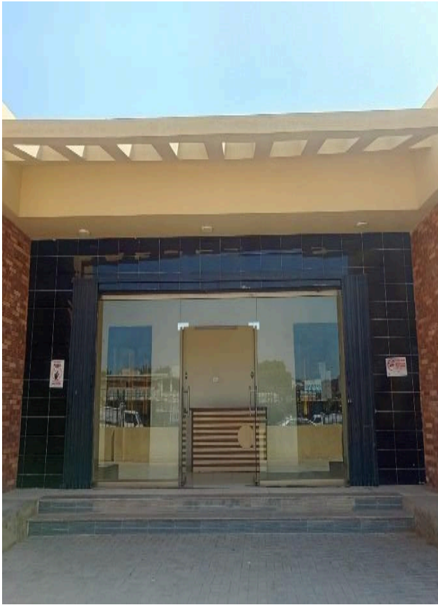
ITC city building
