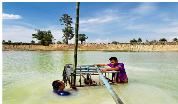
Pond Aeration and Water Circulation System
