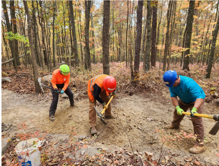
Kate Walker, Paul R. Schmeling and Dan Feer cut sidehill shoulder to shoulder - Photo by Bill Greenan
