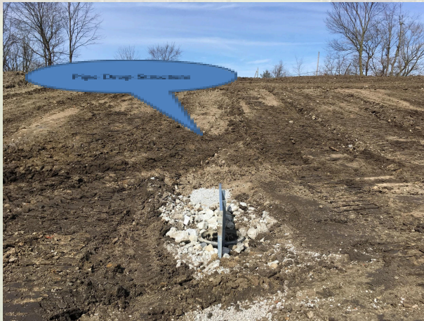
(Dave Burkhart Pipe Drop Structure)
