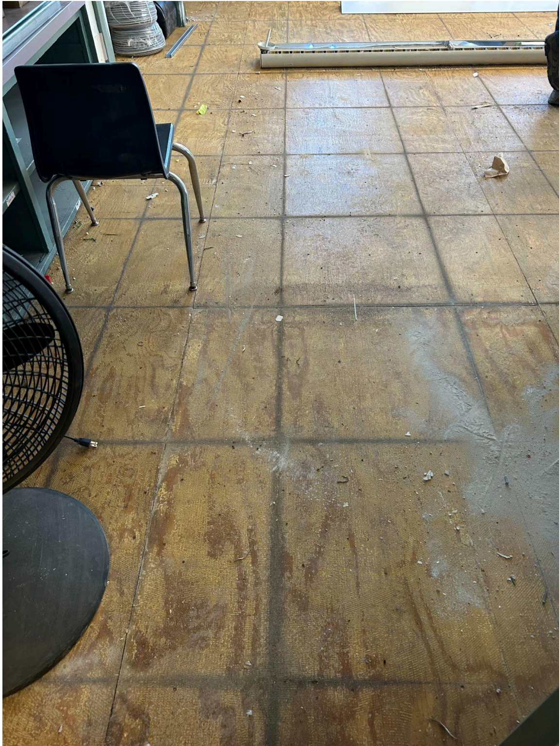
Even the classroom flooring has been removed. There were six workers from Elegant Floors working on site this week, and the entire 1904 wing of the building floors have been completely removed..
