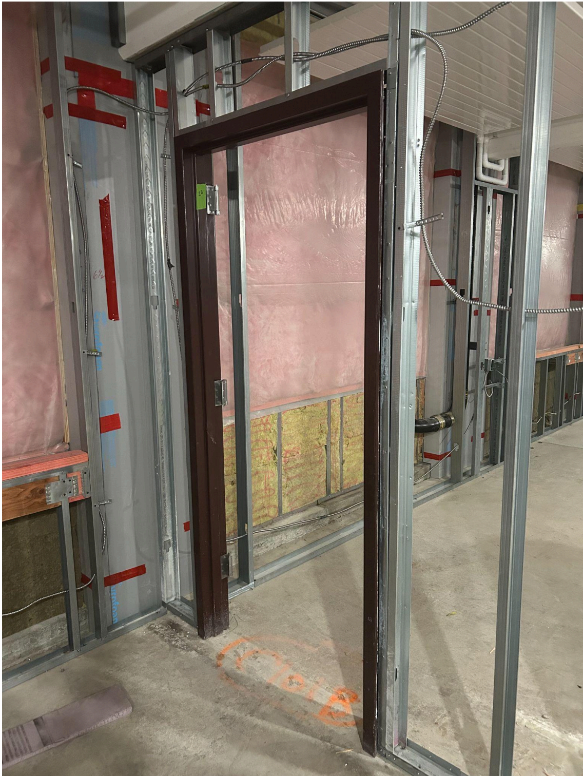
A door frame has been installed in the classroom in the 1965 wing of the building. This door is the door that allows people to go from classroom to classroom without having to go out into the corridor.
